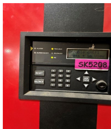
Figures 4 & 5: Expired (2019) fire extinguisher and fire alarm system control pad from 2024 BCFD inspection
