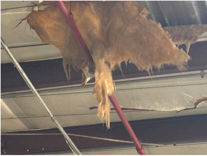
Figures 16&17: Hanging insulation
