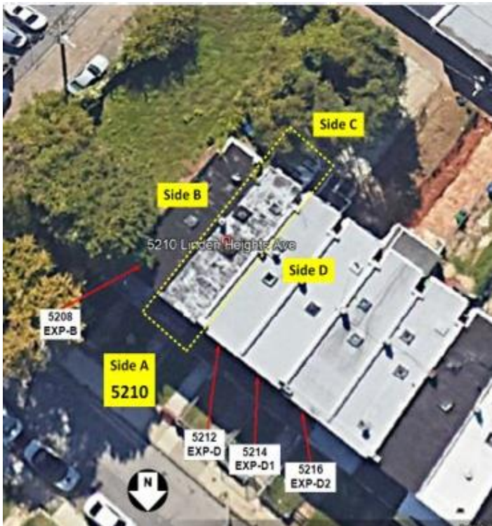
( Photo 2: Pre-fire aerial view of the incident location. Sides of the structure denoted by yellow boxes )
