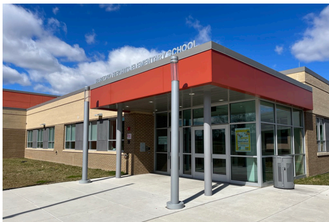
Photo 4. Harford Heights Building (built 1974; renovation/addition completed 2021), 1919 N. Broadway.
