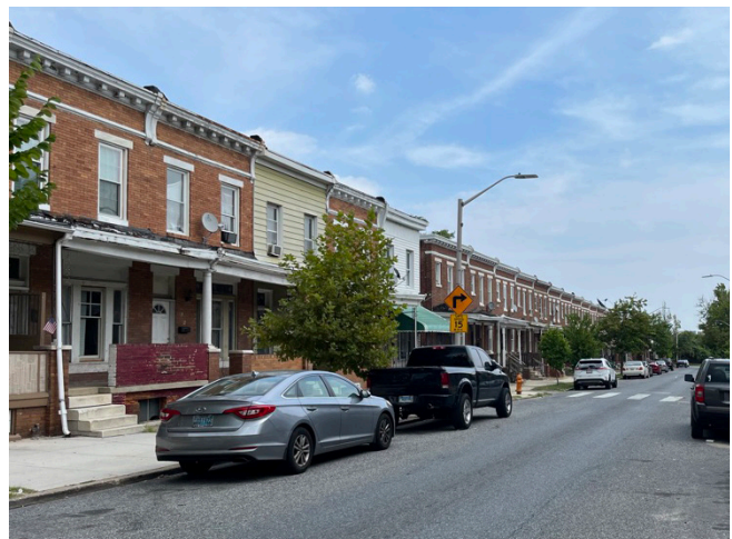
Photo 13. Darley Park rowhouses on the 1600 block of E. 25th Street., 2022 September 30
