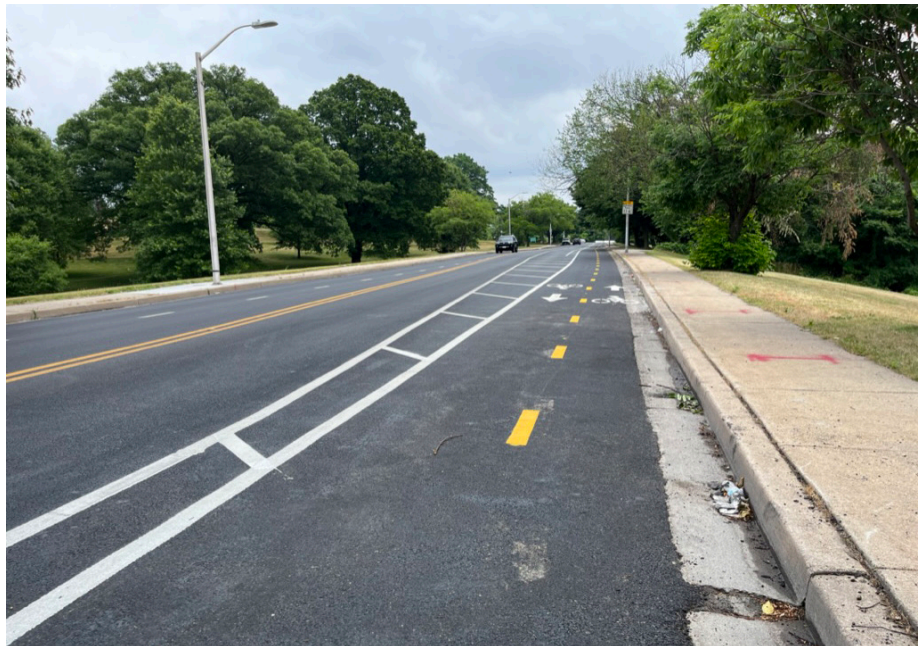
Photo 36. Separated bike lane under construction on St. Lo Drive, 2023 June 12.
