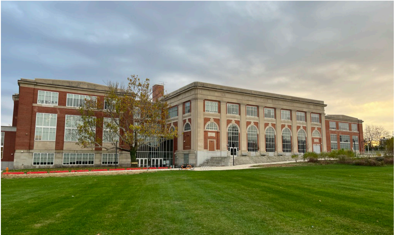
Photo 3. The REACH! Partnership School #341/ Former Clifton Park Junior School (1923; 1922-1924; Josias Pennington, architect), 2555 Harford Road.
