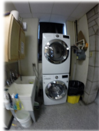
Laundry at back of kitchen
