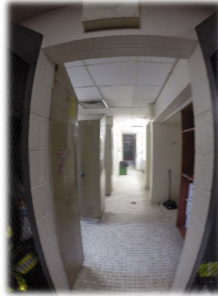
Locker & restroom corridor
