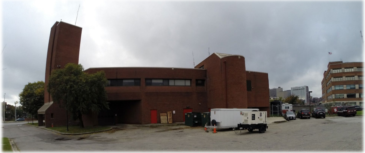
Back of station
