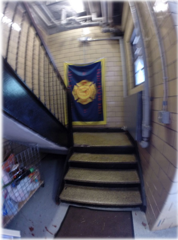
Lower stair landing
