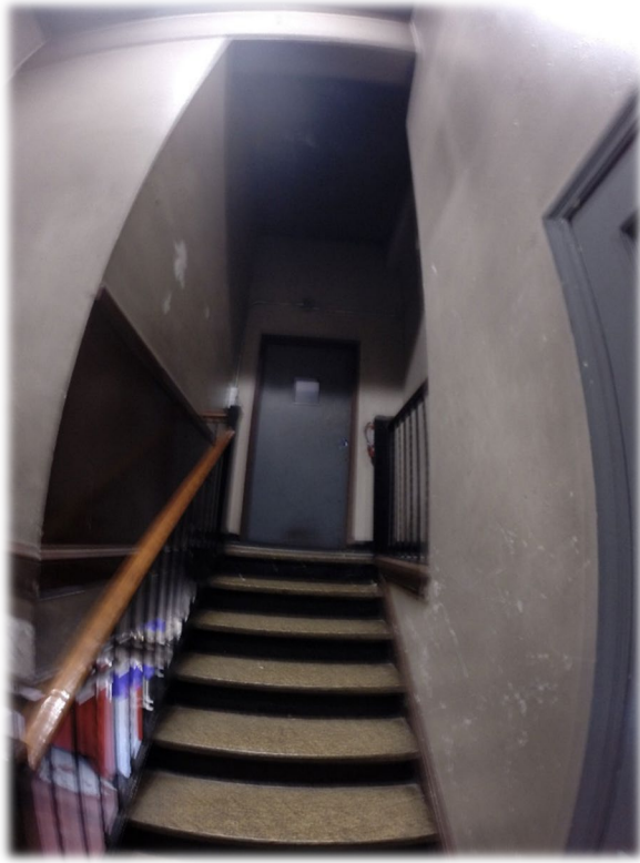
Upper stair landing
