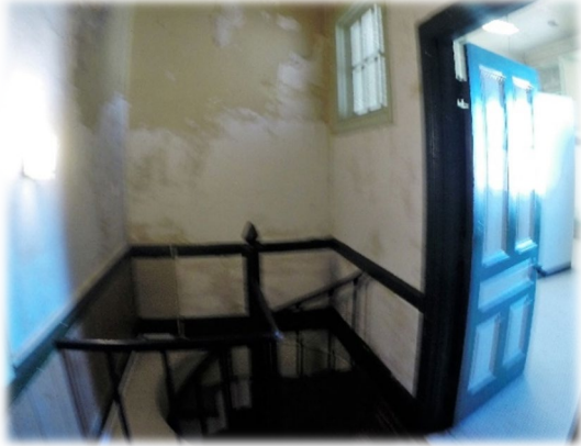
2 nd floor stair landing
