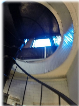
Looking up through stair
