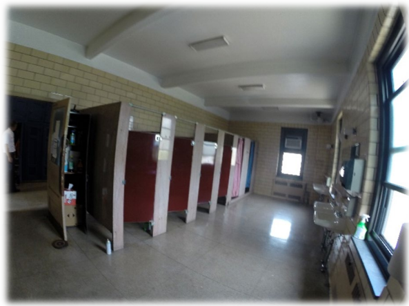
2 nd floor restroom
