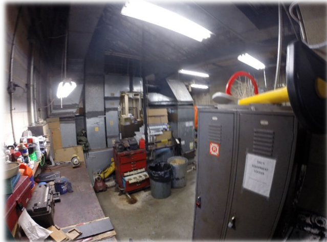
Shop space with electrical equipment
