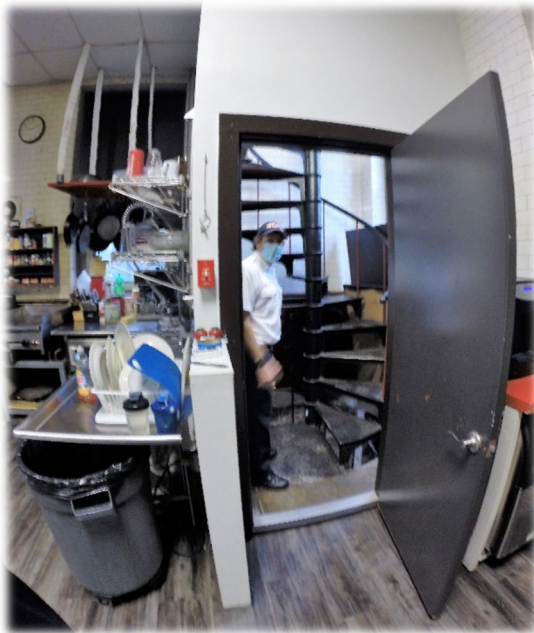
1 st Floor Stair enclosure door
