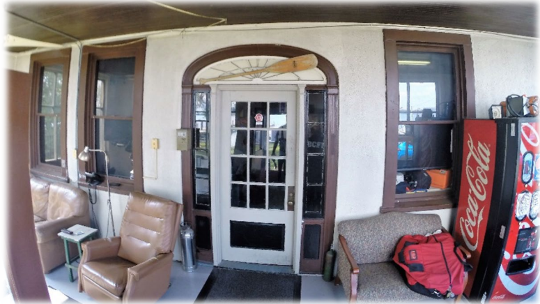
Front door inside front porch
