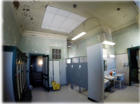
2 nd floor restroom
