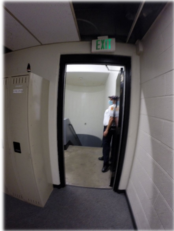
2 nd floor stair landing vestibule
