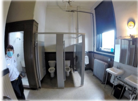
2 nd floor restroom
