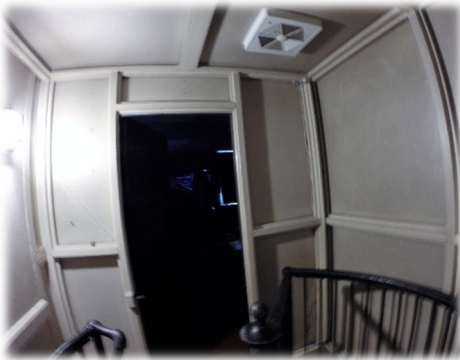
2 nd floor circular stair landing
