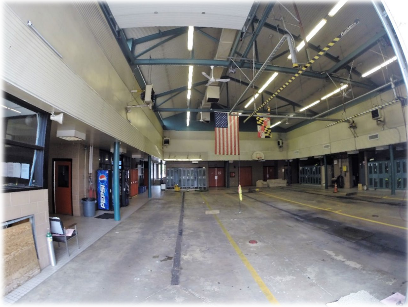
Front looking into bays
