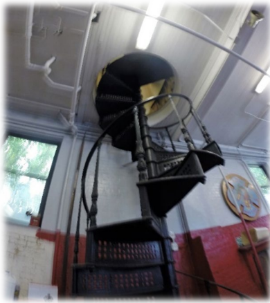
Circular stairs to 2 nd floor spaces
