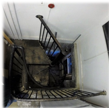
Circular stairs to basement
