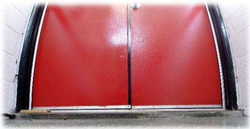
Main exterior doors
