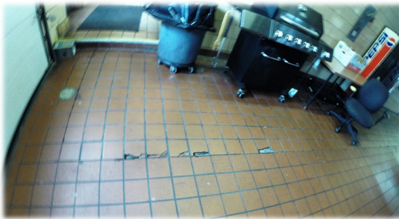
Terra cotta tile bay floor with BBQ and vending machine
