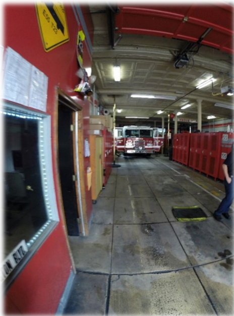
Front of apparatus bay looking back
