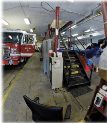
Primary stairs in middle of bays
