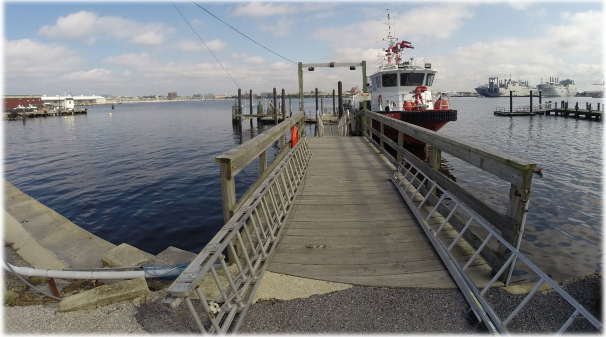
Fire Boat on dock
