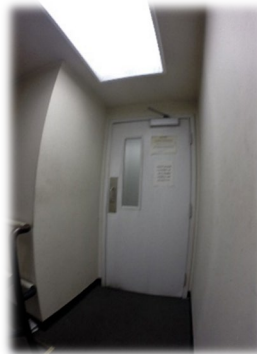
2 nd floor stair landing
