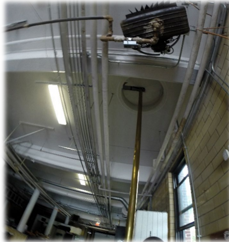
Pole hole with typical plywood "lid"
