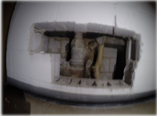
Unfinished repairs to plumbing and electrical
