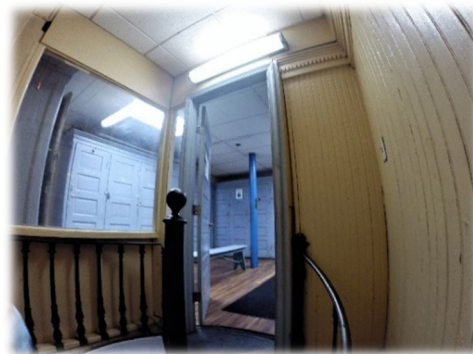
Top of circular stairs
