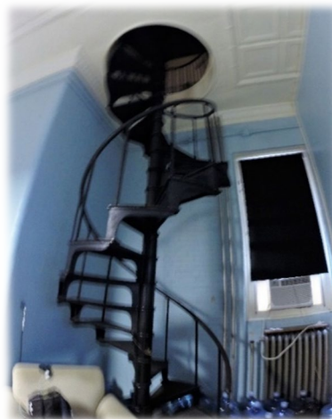
Circular stairs to 2 nd floor
