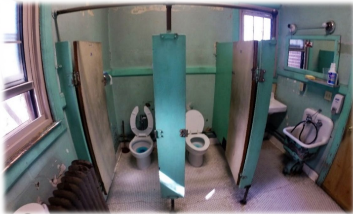
2 nd floor restroom
