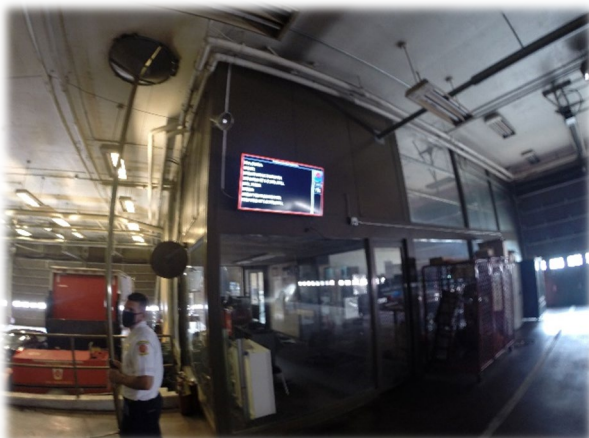
Watch room at intersection of bays
