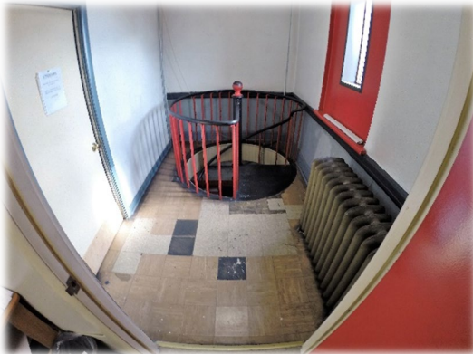
Circular stair landing at 2 nd floor (back of station)
