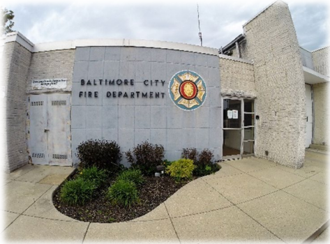
Front door and public entrance
