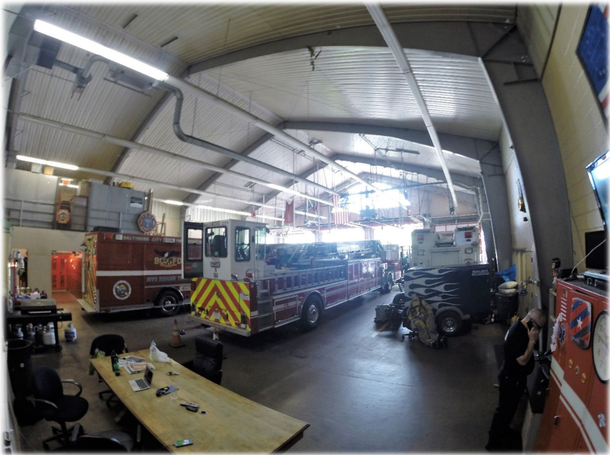
Bay structure is conventional metal building steel frame
