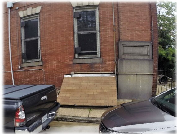
Coal chute has permanent roof
