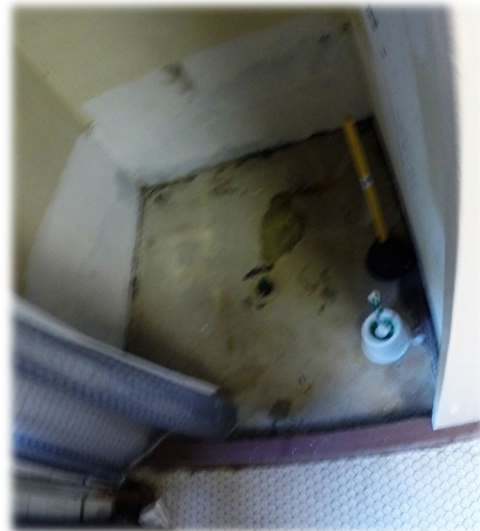
Shower floor repairs
