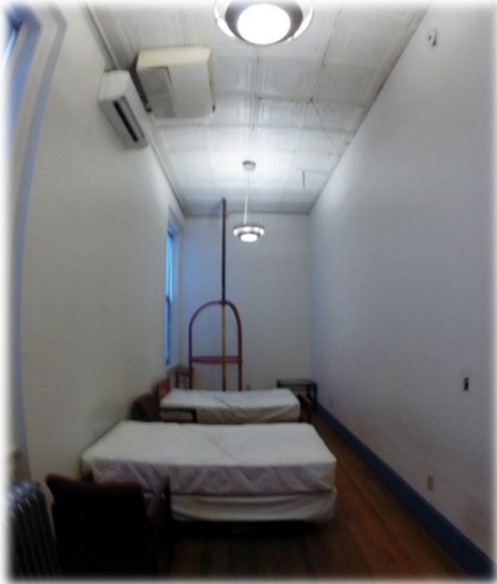
Renovated bunk room with pole access
