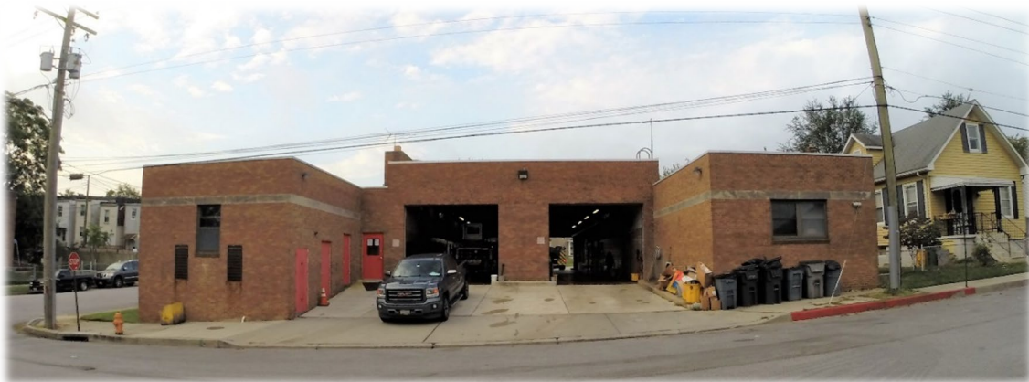
Back of Station 35
