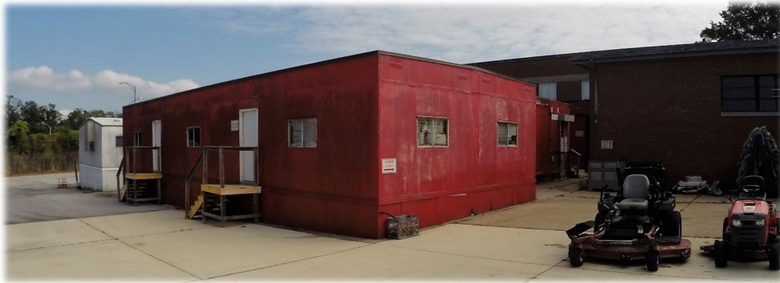
Modular classroom, storage, and locker space
