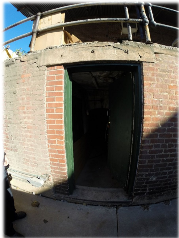
Exterior door to basement
