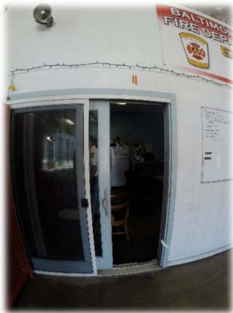
Day room door from bay
