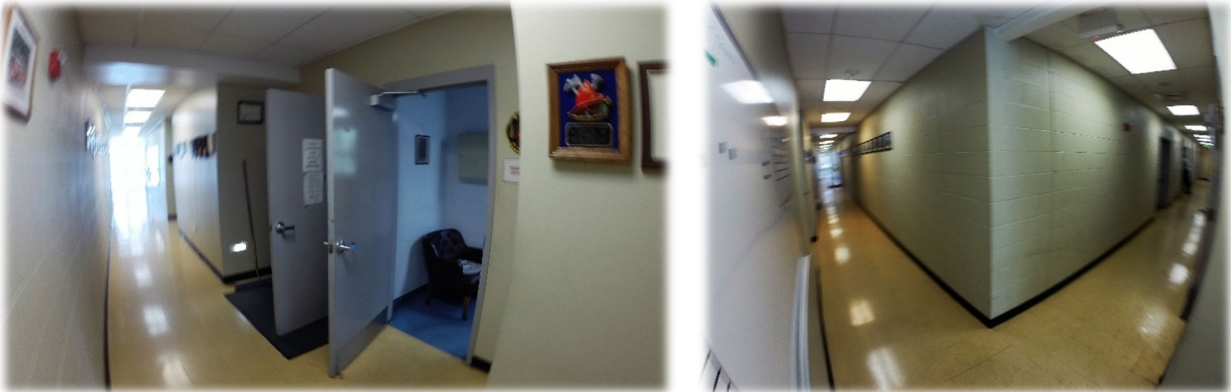
Hallways wrap the apparatus bays and provide access to all living quarters without directly going into bays.
