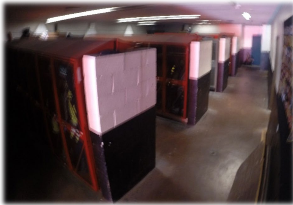
Turnout locker room
