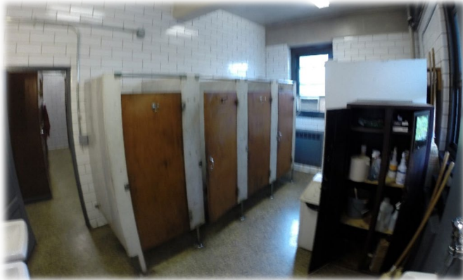
2 nd floor restroom
