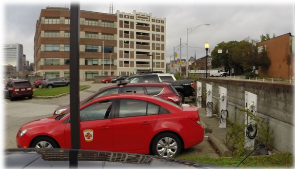
Electric Vehicle charging stations
