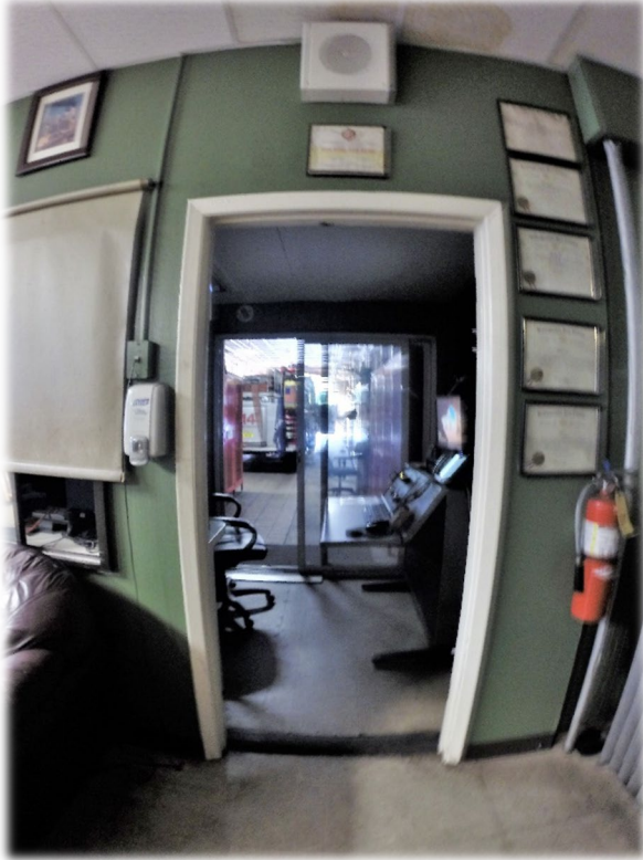
Day room door to watch room and bay beyond
