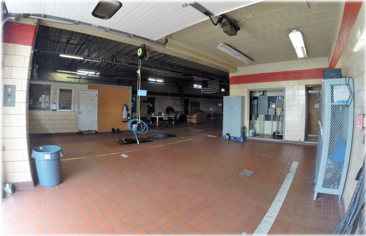
Front of bays looking towards the middle
