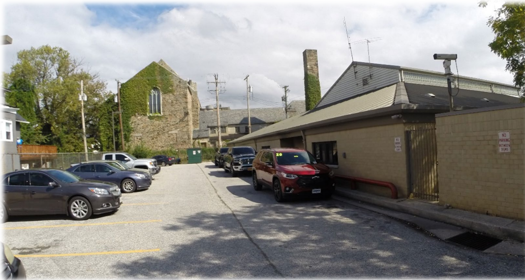
Secure staff parking lot behind station
