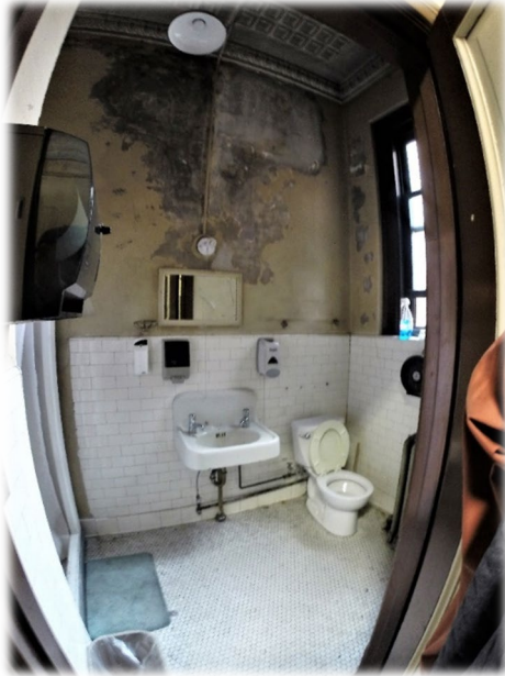
2 nd floor toilet and lavatory
