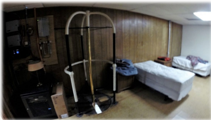
2 nd floor dorm pole hole with typical plywood cover
