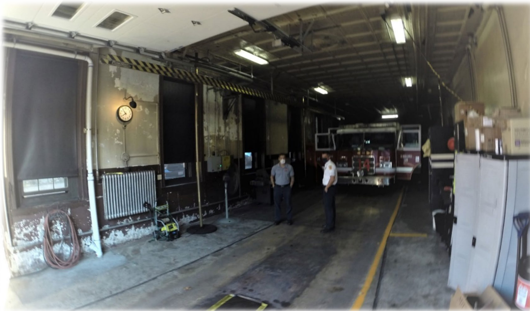
Front of apparatus bay looking towards the back
