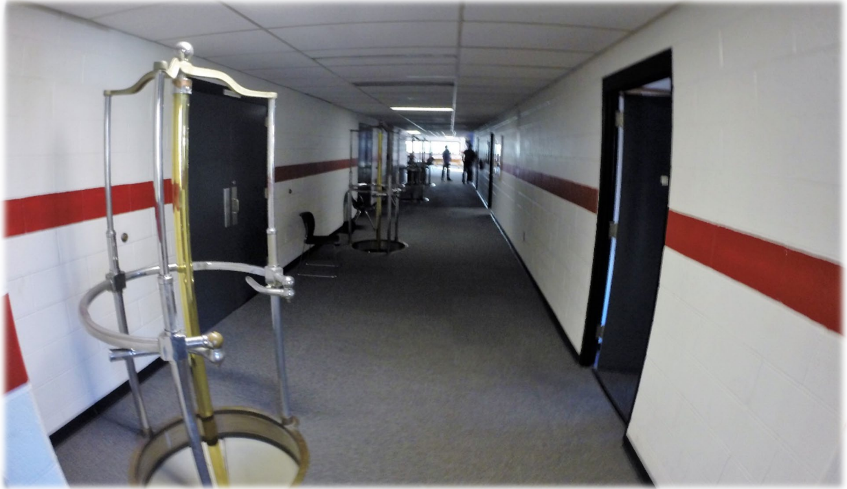
Main hallway and pole holes
