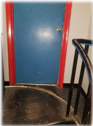
Top of stairs at 2 nd floor
