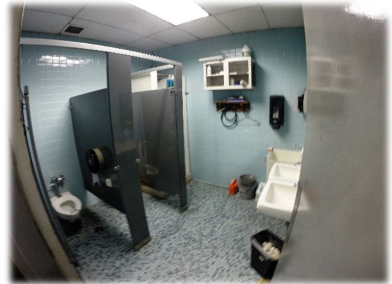
Ground floor restroom
