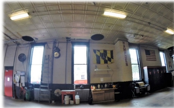
BBQ, abandoned pole holes, and original bell
