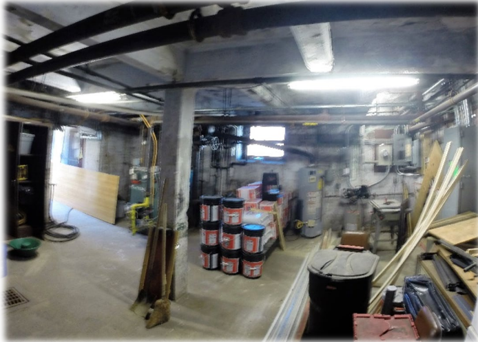
Basement has all utilities and is used for storage
