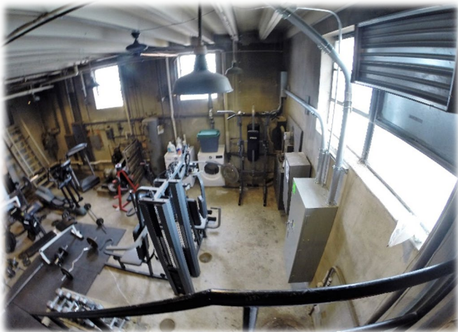
Laundry is in basement behind weights & utilities
