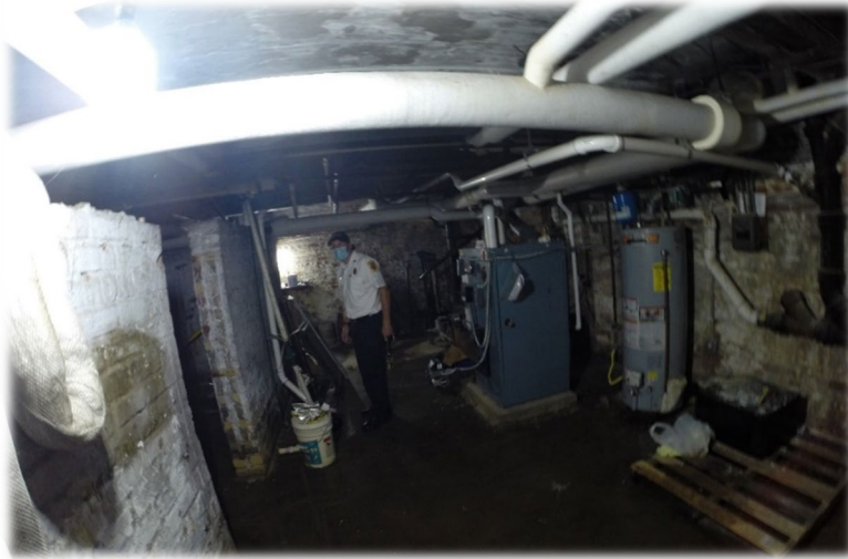
Basement has all utilities and a new furnace and water heater
