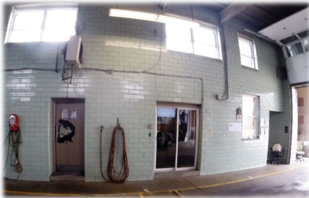
All spaces are accessed directly from bays
