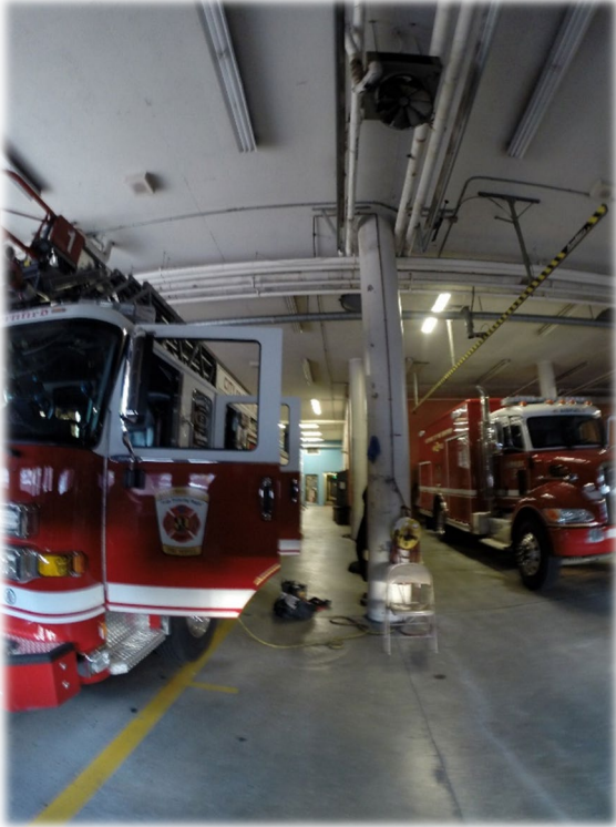
Back of bays
