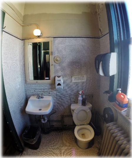
Adjacent restroom renovation
