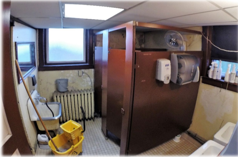
2 nd floor restroom
