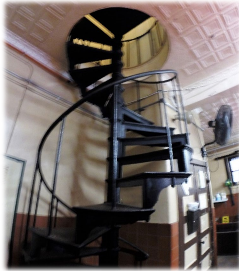
Circular stair at back of bays
