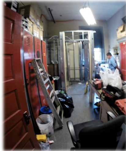
Adjacent restroom renovation
