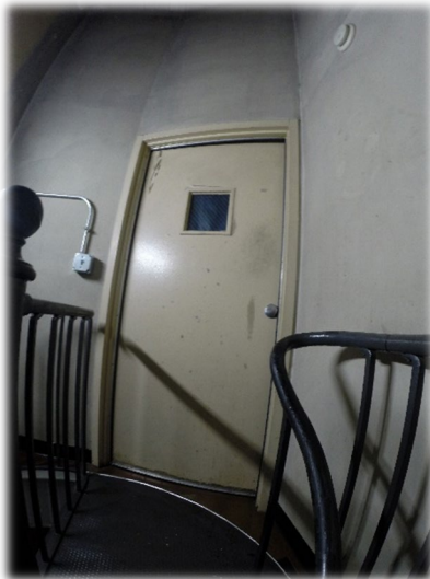
2 nd floor stair landing
