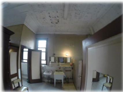
2 nd floor restroom
