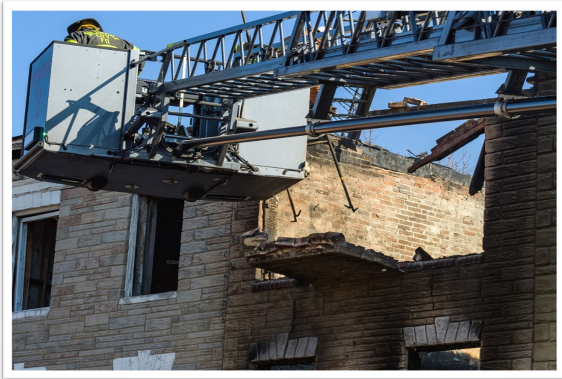
Figure 69 Hooks were used to remove large sections that were cut with saw (Stanley Jaworski)
