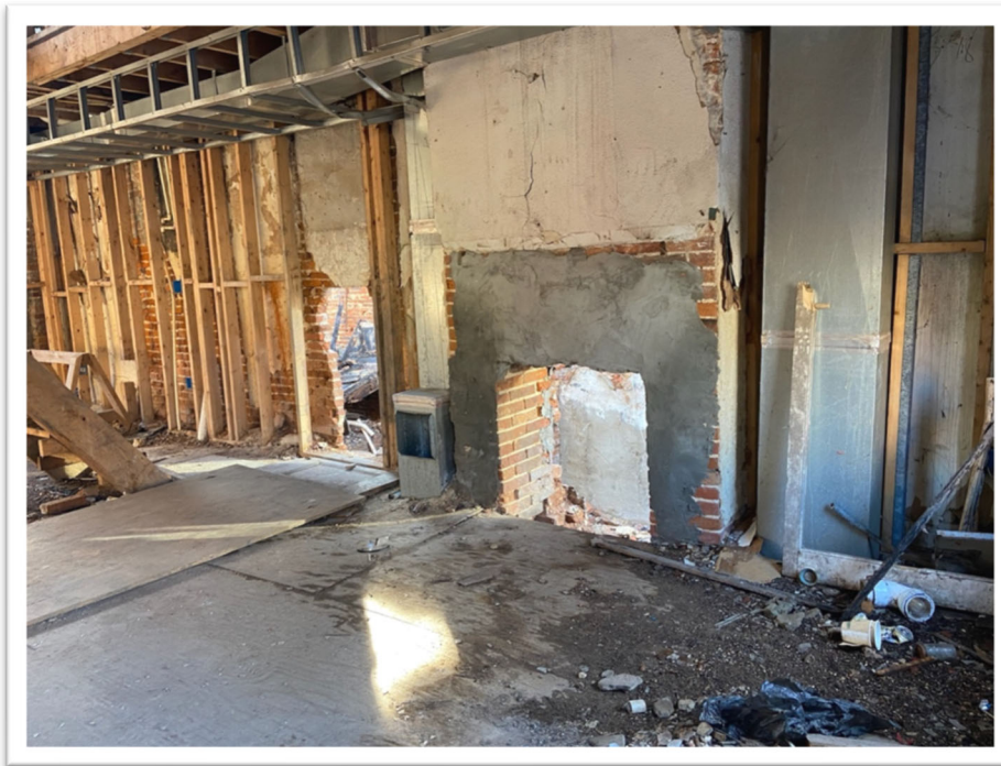
Figure 50 View of breaches from the Bravo exposure (BCFD Member)
