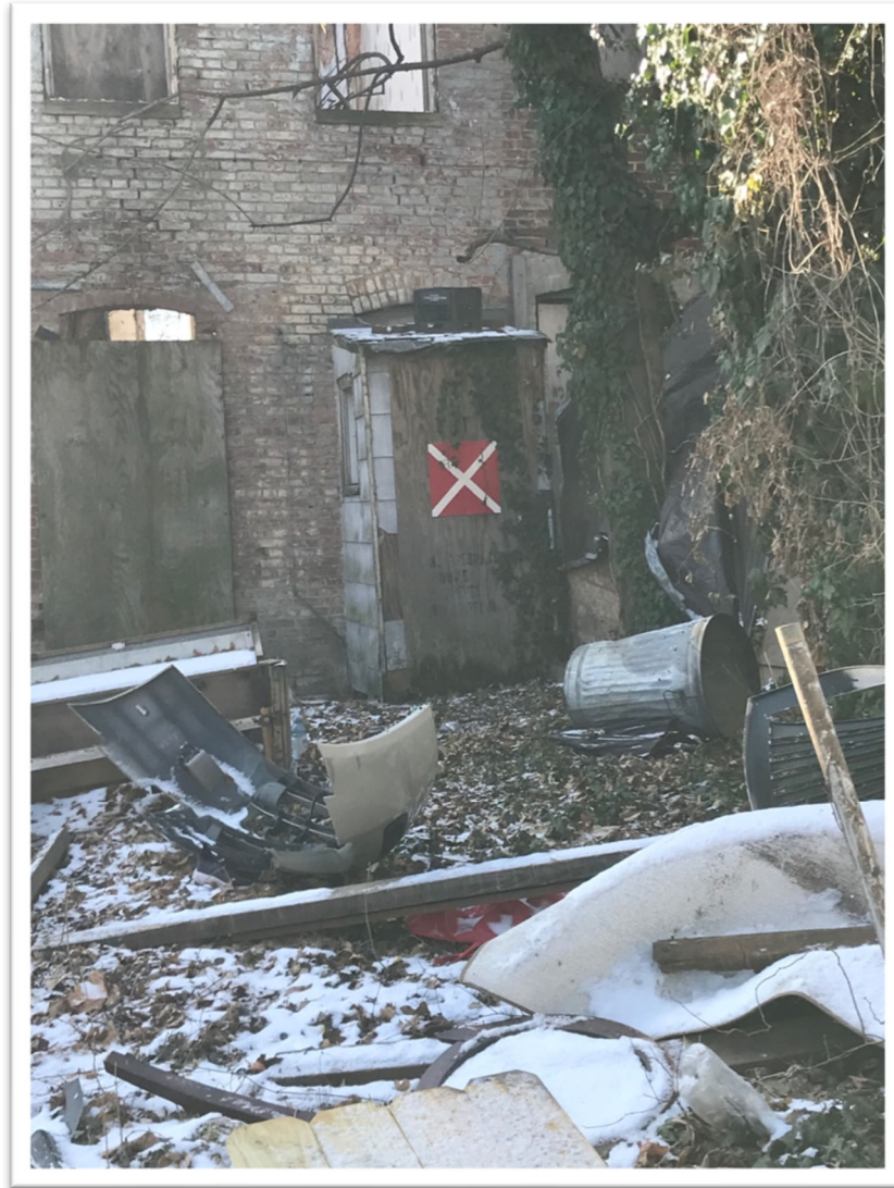
Figure 12 Example of temporary Code X-Ray placard attached to the rear of a dwelling (BCFD Member)
