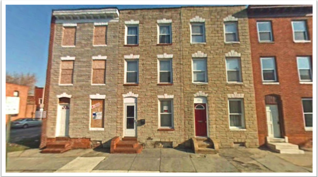
Figure 24 205 South Stricker Street December 2007 (Google Maps)
