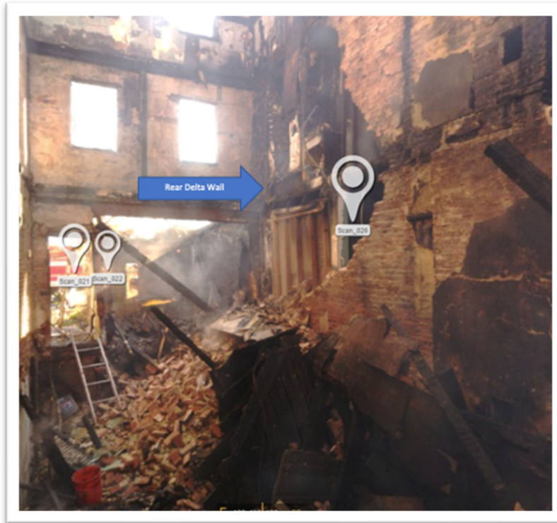
Figure 65 The rear Delta Side party wall after secondary collapse looking in from front door on Side Alpha (ATF)
