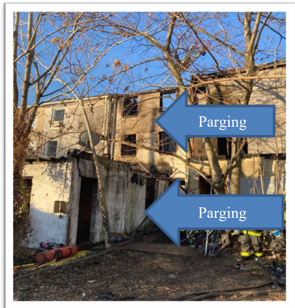
Figure 22 Side Charlie brick façade with cement parging (FIB)
