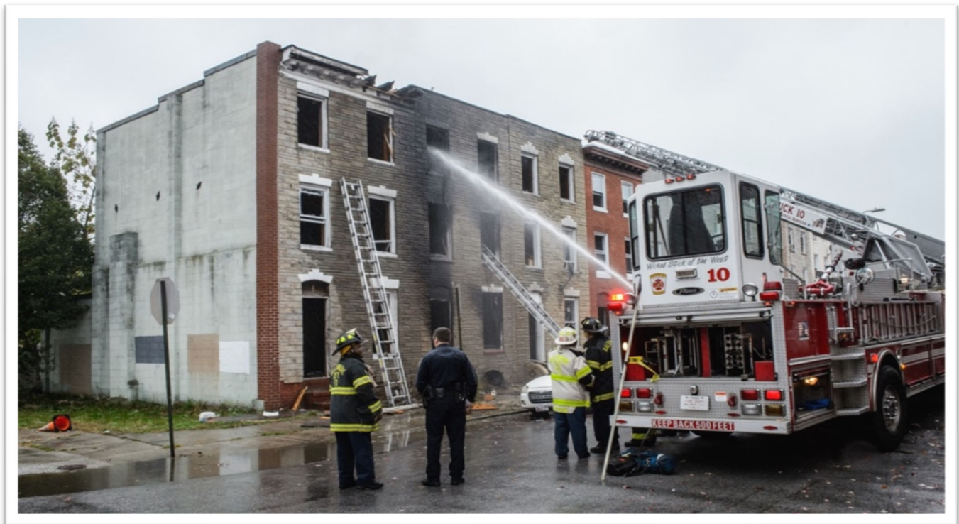
Figure 27 Fire Building after fire in October 2015 (Stanley Jaworski)
