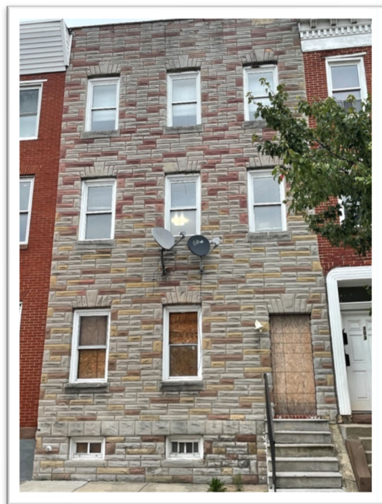
Figure 4 Appears vacant but is occupied (BOI)
