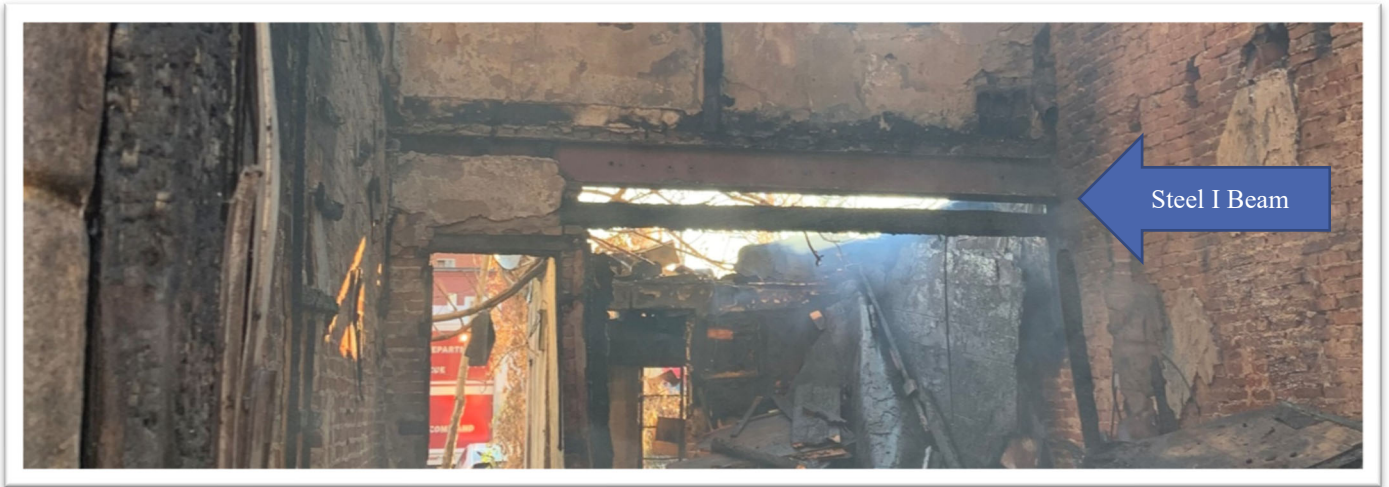
Figure 18 Steel I-beam running across Charlie Side rear wall (FIB)
