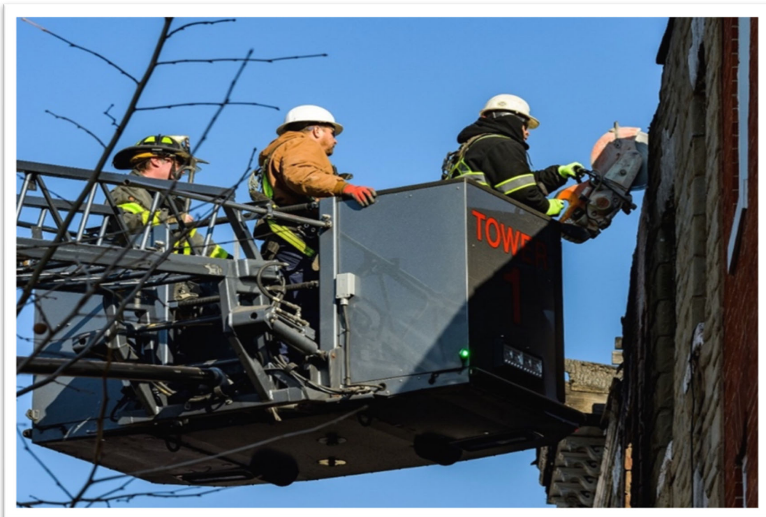
Figure 68 Contractors working on cutting through bricks on Side Alpha (Stanley Jaworski)
