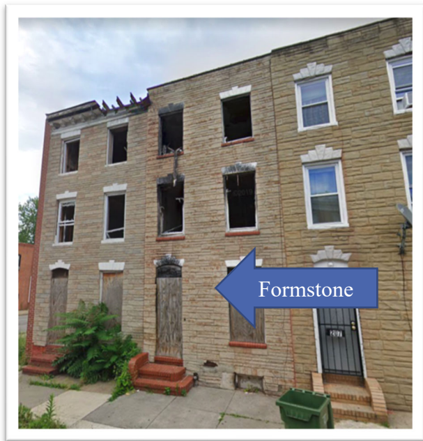
Figure 21 Side Alpha brick façade with a Formstone covering (Google Maps)
