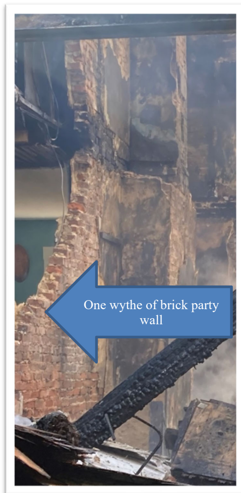
Figure 19 One wythe party wall separating the adjacent structures (FIB)
