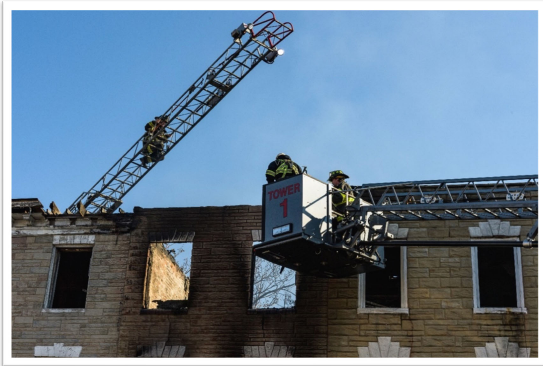
Figure 67 Tower 1 in position to assist with removal of Side Alpha while. Member was positioned on the aerial of Truck 16 as another set of eyes (Stanley Jaworski)
