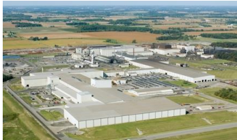
Butler, IN Greenfield EAF Steel Mill • 3.2M Tons • 3 Galvanizing Lines • 2 Paint Lines
