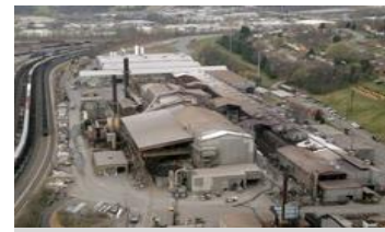
Roanoke, VA Acquired/Expanded EAF Steel Mill • 720K Tons • Merchant and Rebar
