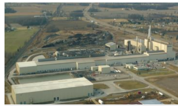
Pittsboro, IN Acquired/Expanded EAF Steel Mill • 950K Tons • Special-bar-quality • Value-Added Finishing/Inspection Lines
