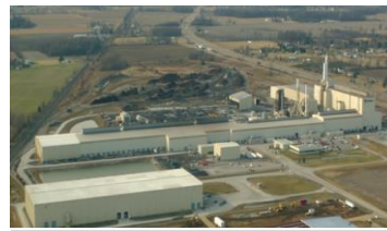
Pittsboro, IN Acquired/Expanded EAF Steel Mill • 950K Tons • Special-bar-quality • Value-Added Finishing/Inspection Lines
