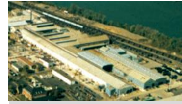
Huntington, WV Acquired/Expanded EAF Steel Mill • 580K Tons • Specialty Shapes
