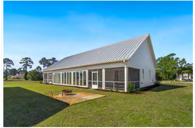
Firepit area, plumbed for summer kitchen
