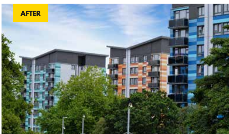
RECLADDING CHARLEMONT FARM ESTATE, UK.
