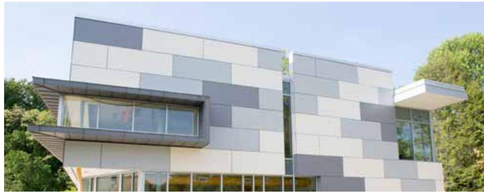
future, Renfrow needed to find a durable material that could withstand time and weather, while fulfilling LEED Gold sustainability requirements, as well as aesthetic and budget requirements. Renfrow's research pointed to ventilated façades, commonly used in Europe, and as a result high quality Trespa® Meteon® panels were selected.
