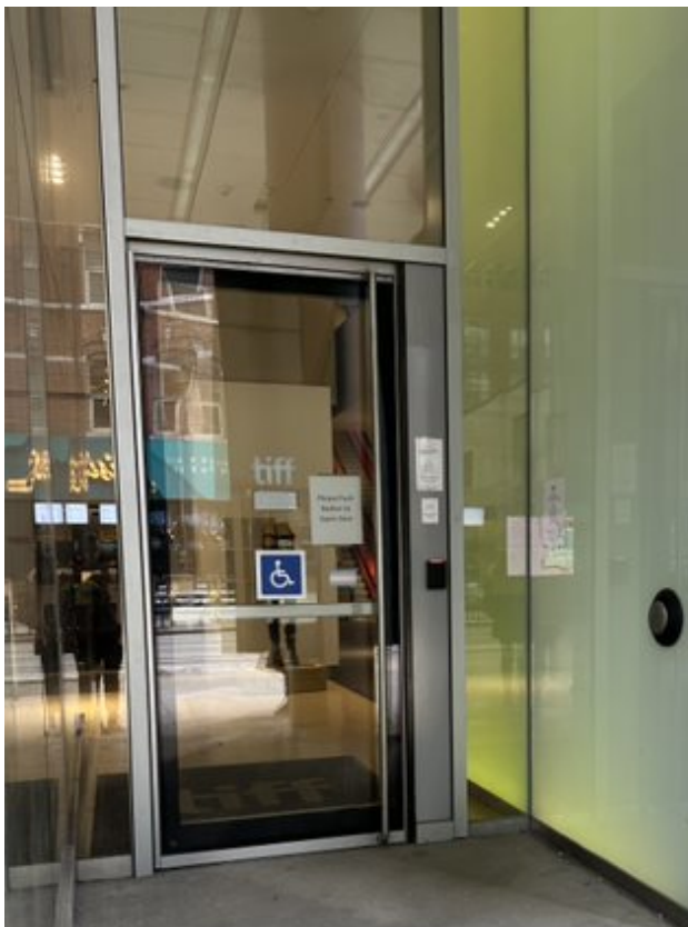
Accessible doors at Main Entrance
