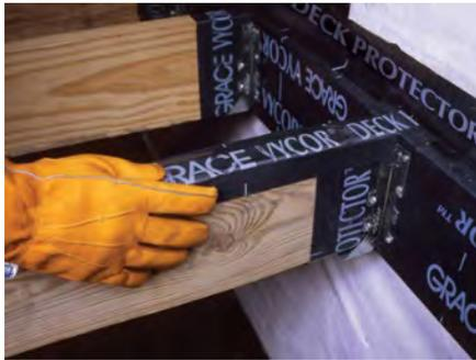
Fiberon also recommends spacing the joists at 12 in. on-center to increase stability and reduce the flexing of the deck boards. This will also help to minimize potential noise.
