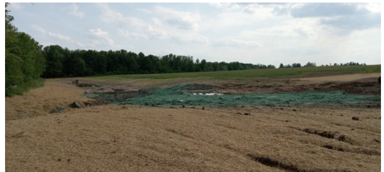
After photo of the Pork Street wetlands project with seed and mulch cover applied. Credit: Onondaga County Soil & Water
