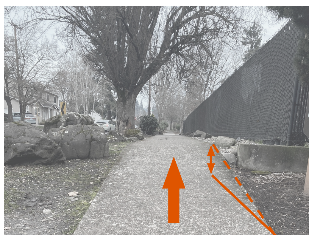
Running Slope , or grade, is in the direction of travel.
