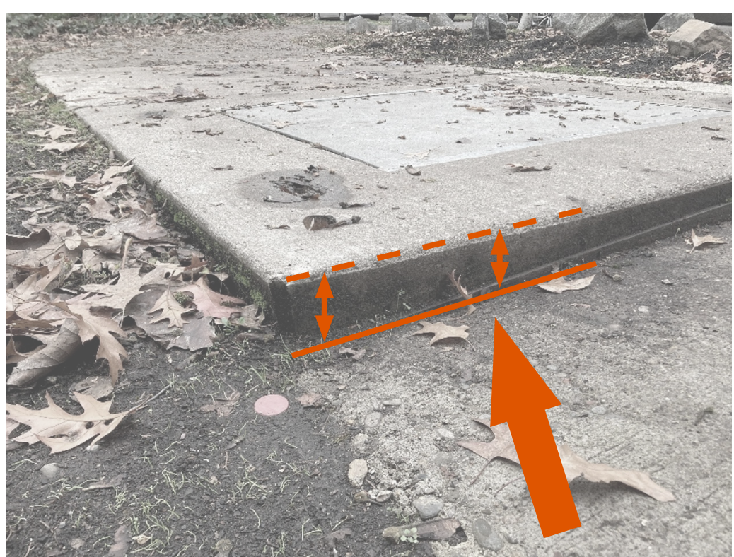
Uplift is a height difference where two pavers meet.
