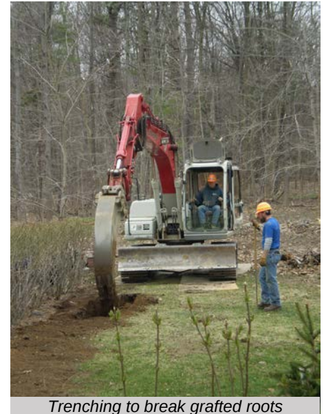
Trenching to break grafted roots
