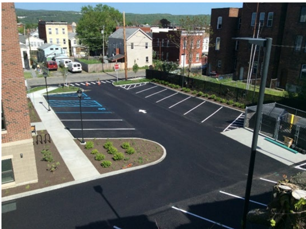
Porous Asphalt parking stalls installed in Cohoes, NY
