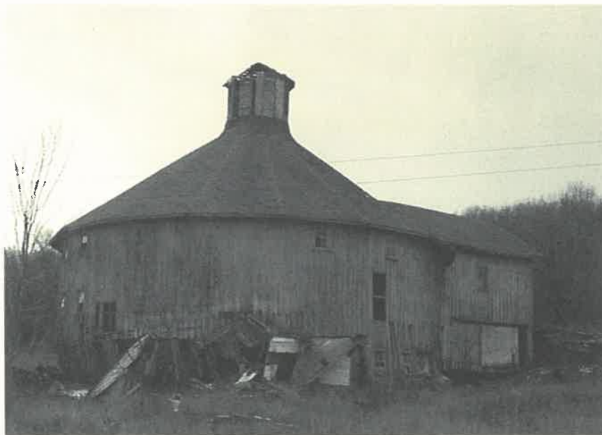
Round Barn - Pines Brook Road, Walton (Delaware County). In poor state of repair - entrance to bay storage by ramp. Cows housed in basement - heads faced in towards central hay storage.
