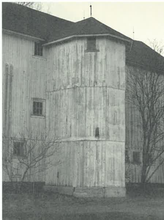
Hidden Silo - Two 16' x 16' square silos are hidden in the end of this barn. Rice Homestead.
