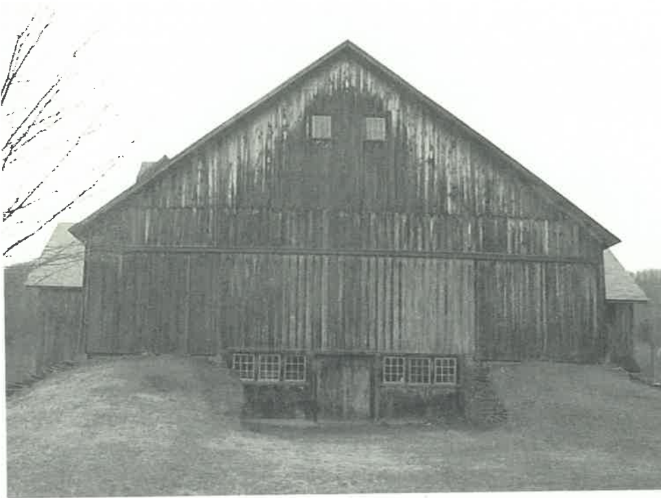
On Grade - Tyler Barn, Walton, NY (Delaware County). Barn built on grade with double earthen and stone ramp to 2nd floor.
