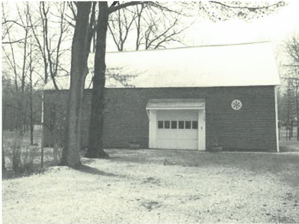
Restored Dutch Barn - raised a few feet, doors moved to sides, evidence of gable end doors visible on inside. Village of Middleburg, River Street.
