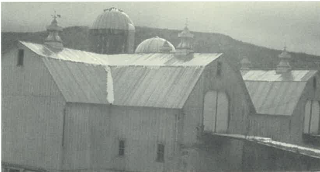
Lamport's double ramp barn with gambrel roof and multiple ventilators. Route 10, Stamford, NY (across from McMurdy Brook Road) (Delaware County)
