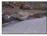
**Exposed stock piles and soil** can easily run off construction sites resulting in costly repairs clogging drainage structures.
