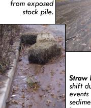
Straw bales can easily shift during storm events allowing sediment to enter nearby stormdrains.
