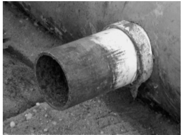
*Figure 4 – Four inch nipple in trunkline*
