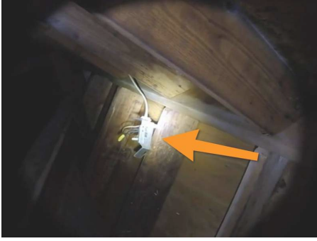
Attic over northwest BR
