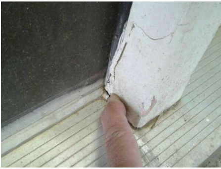
Lower level kitchen door
