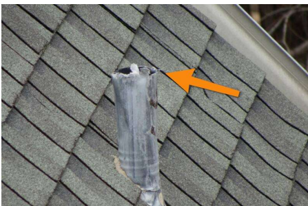
East side upper roof
