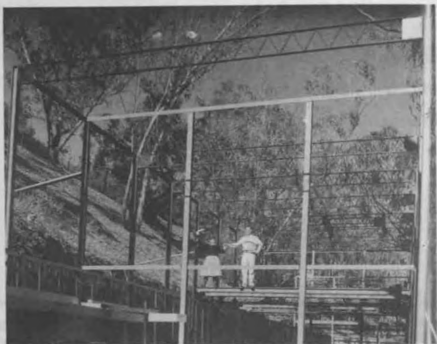
Figure 15.1. Ray and Charles Eames on the newly constructed steel frame of their house in Pacific Palisades, California, 1949. Library of Congress, Prints and Photographs Division. Copyright Lucia Eames/Eames Office ( www.eamesoffice.com ).
