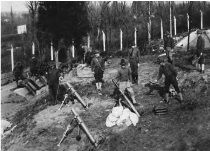
Figure 9.14 Mortars were used to fire large quantities of shells into the woods and fields near the Potomac River to test the shell fuzes and the spread of the gas. The cement angular Livens mortar platform on the left side of the photo found by Terry Slonecker, Greg Neilson, and the author, allowed the mortar range fan to be accurately determined. Several live shells were recovered from the mortar fan.
