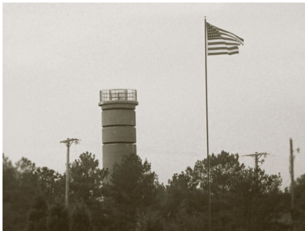
Figure 10.22 Fire control tower from Cape Delaware.
