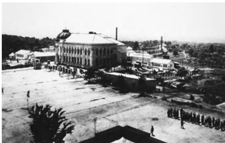
Figure 9.9 Haber nitrogen fixation furnaces (one under construction) in rear (1917–1918). These ran twenty-four seven making large quantities of nitrogen used for explosives.
