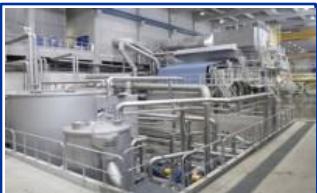
Indonesia – Installation, pre-com/commissioning of Pelita Cengkareng paper mill gas turbine generators
