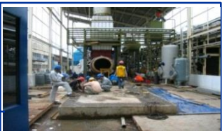
Indonesia – Installation, pre-com/commissioning of Bridgestone type manufacturing plant gas turbine generators
