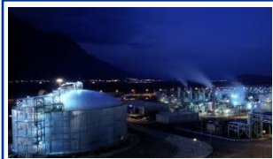
Iran – Warranty survey and initial inspection for KPIC petrochemical plant gas turbine generators
