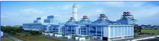
Singapore – Installation & pre-commissioning of NFL co-generation plant gas turbine generators
