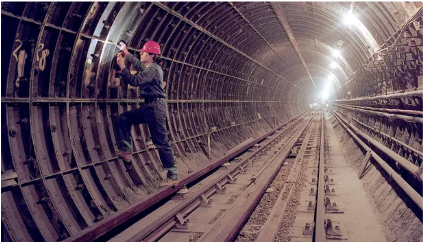
A worker inspects segmental tunnel lining under Angel Underground station, London (Credit: Jim Byrne/Getty)
