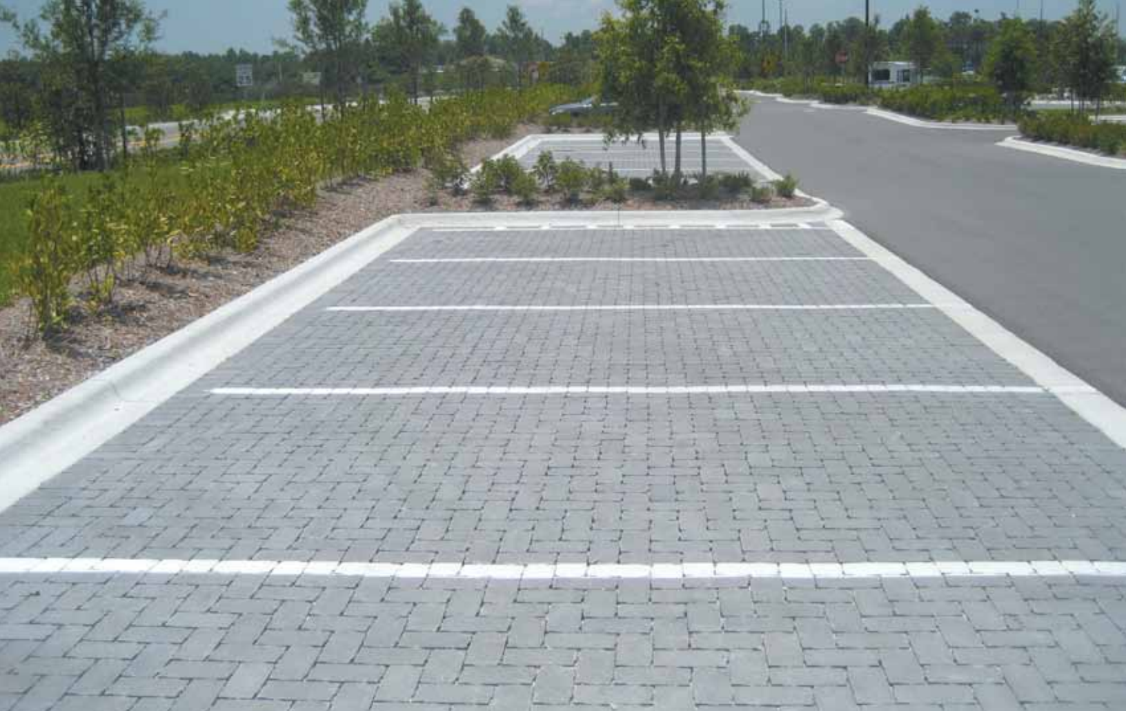
Project: Walmart, Location: Tampa, Florida
