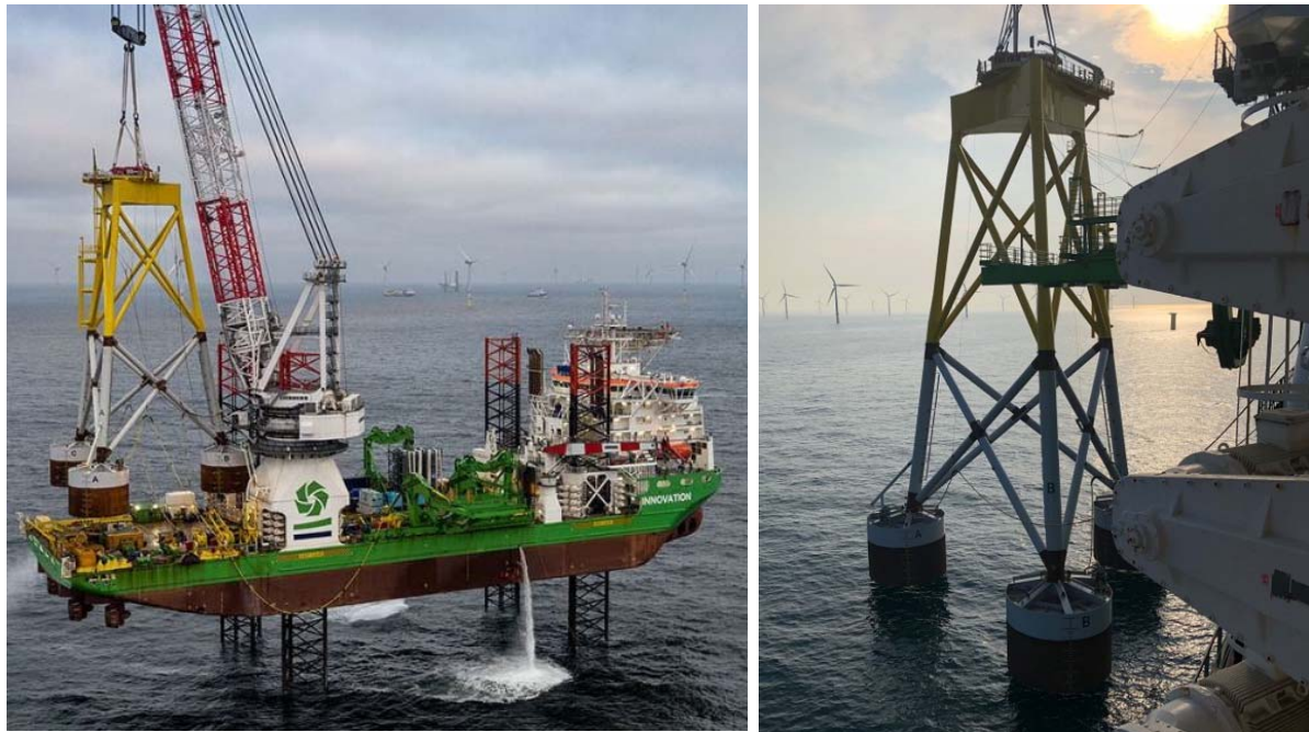
Figure 1 Photos of the Borkum Riffgrund 2 suction bucket jacket installation
