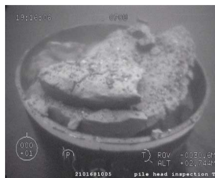
Fig.1. Residue from soil plug in pile (stick-up: 2.4 m) after excessive efforts to remove follower
