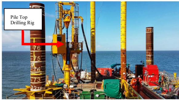
[i] Pile top drilling rig on Conductor Pile A1
