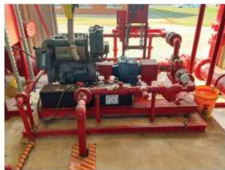
The facility operator agreed to GST's recommendation that PFAS-SOL be deployed to reduce the concentrations of PFAS residues on the fire-fighting system piping and equipment surfaces.
