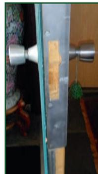
Steel plates on door edges and door service bolts (right) prevent doors from being kicked in.
