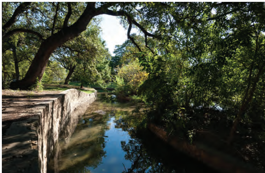
Acequia Madre Mission de Valero, Bexar County, Texas. The Spanish and their Indian charges built this irrigation ditch (acequia) after the founding of San Antonio in 1718. Hand dug and made of dressed limestone, the acequia diverted water from San Antonio River through agricultural fields that belonged to San Antonio de Valero Mission. Credit: photo by Christopher Talbot, National Park Service
