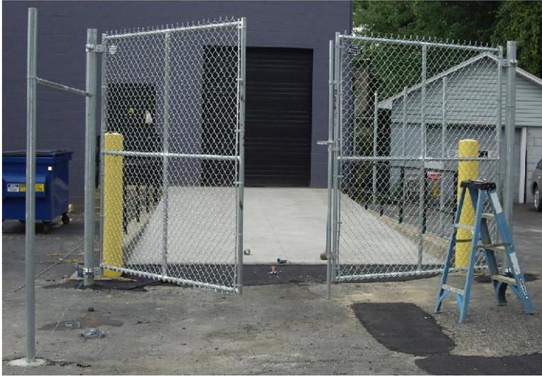
2. Three Way + Tie In. There may be more than one fence line tying into the posts. Thus, requiring additional post height to accommodate all the end bands.
