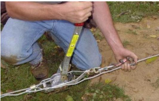
5. Make sure that you leave at least a one foot section to wrap around the wire. Tension wire is
