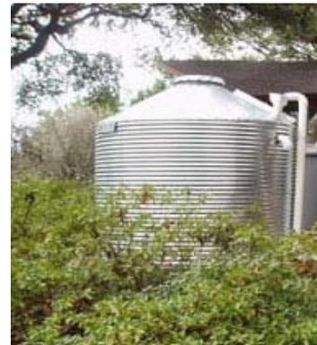
These tanks are for above-ground use. Old or recycled tanks may contain lead and should be avoided. Brass and bronze fittings should not be connected directly to the tank as they will cause corrosion. Additionally, care should be taken when cleaning
