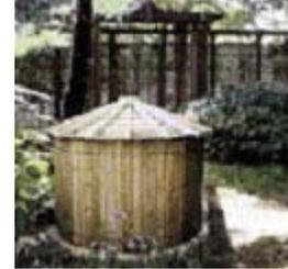
Redwood, as a tank material, has a great reputation for being durable and attractive. It contains no resins and has high levels of tannin, a natural preservative resistant to insects and decay. It is also a good insulator, keeping the water cooler in the summer and protects it from freezing the winter.
