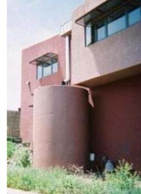
One unique advantage of poured concrete is that the concrete will over time decrease the corrosiveness of rainwater by leaching into the water. This advantage of concrete tanks results in a desirable taste imparted to the water by calcium in the concrete being dissolved in locations where there is slightly acidic rainwater. For potable systems, it is essential that the interior of the tank be plastered with a high-quality material approved for potable use.
