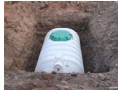
Polyethylene tanks tend not to retain paint well, so use pre-painted (i.e. pigmented) tanks manufactured with opaque plastic. Black and dark colored tanks will absorb heat and thus, should be shaded or buried. The fittings of these tanks are aftermarket modifications and are easy to plumb. However, the fittings are not always tight, and should be checked for leakage occasionally.
