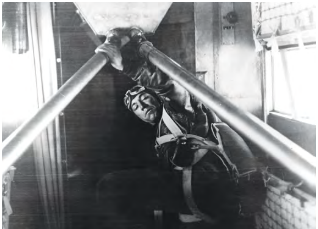
Lt. Elwood Quesada adjusts an aircraft gas line during a 1929 operation dubbed Question Mark where a 10,000-pound Fokker C-2A was refueled in flight by two modified Douglas C-1 transport aircraft. (Archive photo).
