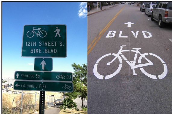
Bicycle Boulevard Signage and Pavement Markings.
