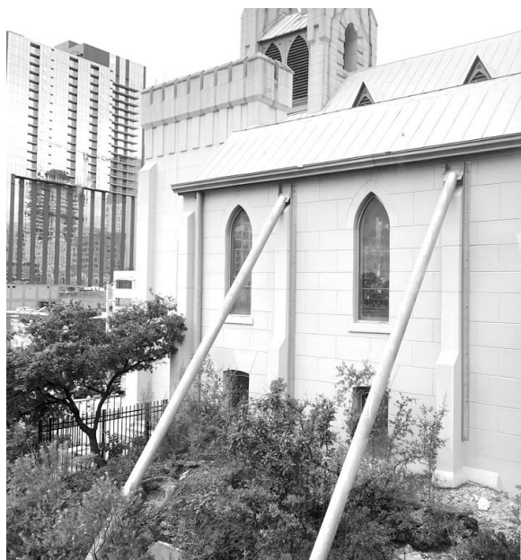
East side braces were installed in 2016 to help stabilize west wall. Eric Leibrock
