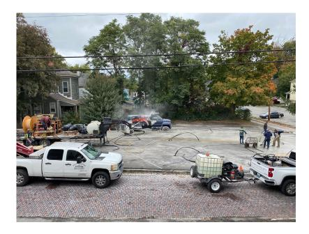
Next they'll dig small trenches in order to be able to connect the pipes between each hole, so that each well is connected to the next one and we end up with one continuous loop. They'll also run a pipe beneath the brick alley so that the loops of pipes can be connected to gear that will be installed inside the church basement.
