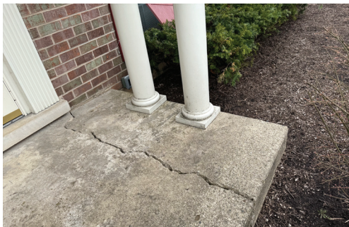
Damage to the front stoop
