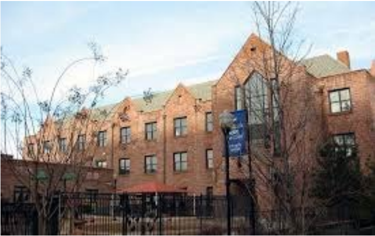
Building Pritchett Center
