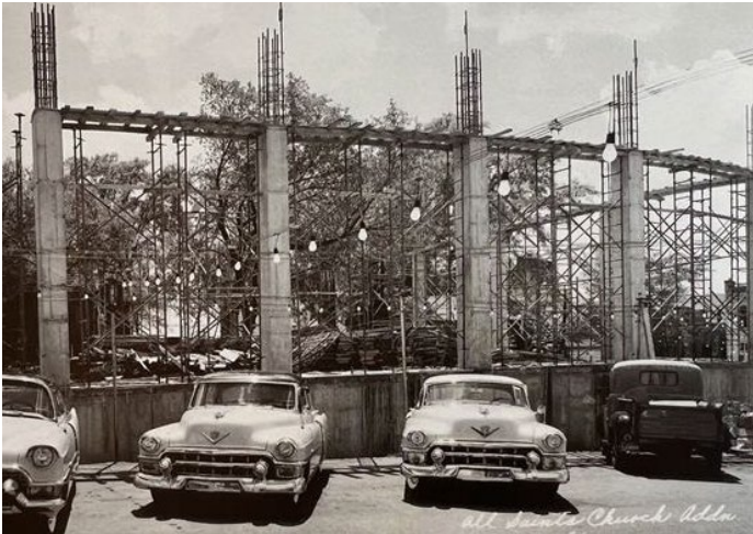
Parish House construction, 1956
