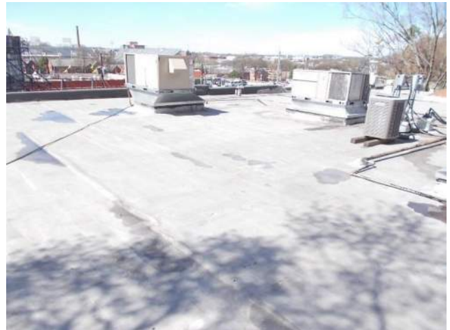
Figure 6.3-4. View of the main lower roof area from the northwest and southeast corner of the roof.
