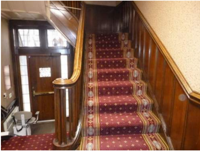
Figure 3.3-7. Overall view of a wood framed stair at the second floor.
