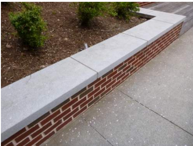
Figure 7.3-7. Partial view of a site wall at the Kennedy Commons Courtyard.
