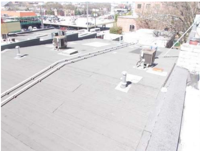
Figure 6.2D-3. Overall view of the roof area.
