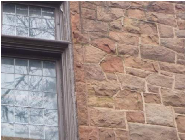
Figure 3.2-1. View of brown sandstone on the exterior of the Egleston building.
