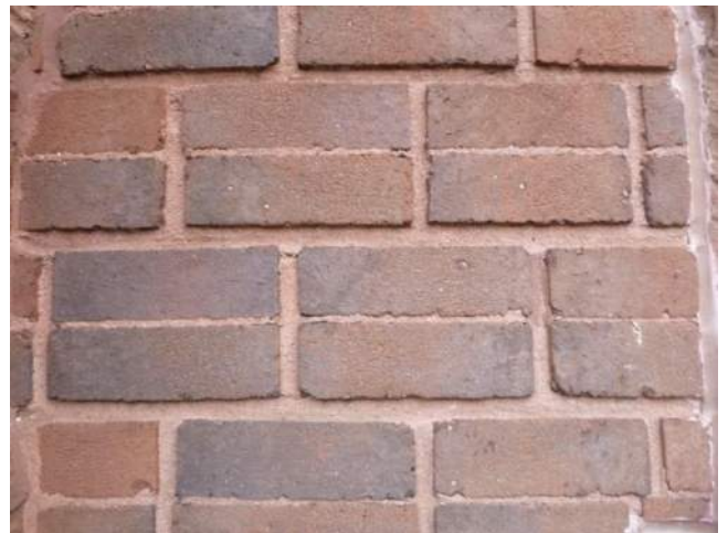
Figure 3.2-10. View of an area of typical block bond masonry on the Egleston building facade.
