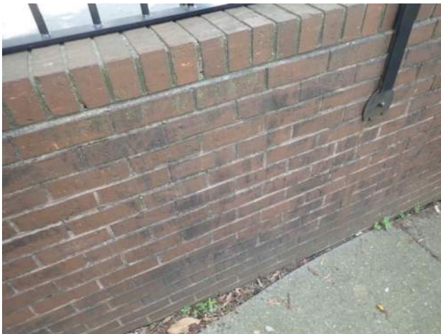
Figure 7.3-1. View of a brick masonry site wall and fencing.
