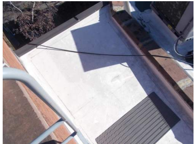
Figure 3.1-2. Overall view of the north end of the lower roof from the top of the east parapet wall of the Parish House roof.
