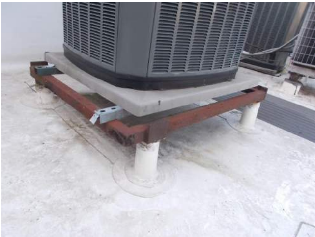
Figure 3.1-17. Equipment supports integrated with the roofing assembly.
