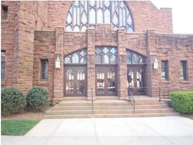
Figure 2.2-25. Wood entrance doors at the east facade of the Church were in good condition.
