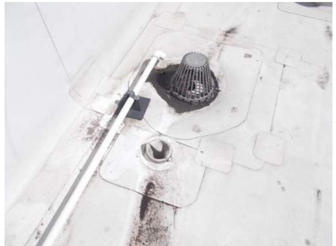
Figure 5.1-24. No drain grates or covers were provided on the overflow drains.
