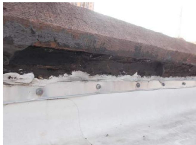
Figure 3.1-20. Mechanically fastened termination bar that is sealed with sealant.
