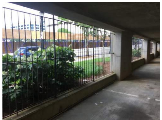
Figure 5.3-6. View of metal fencing between openings in the parking structure.
