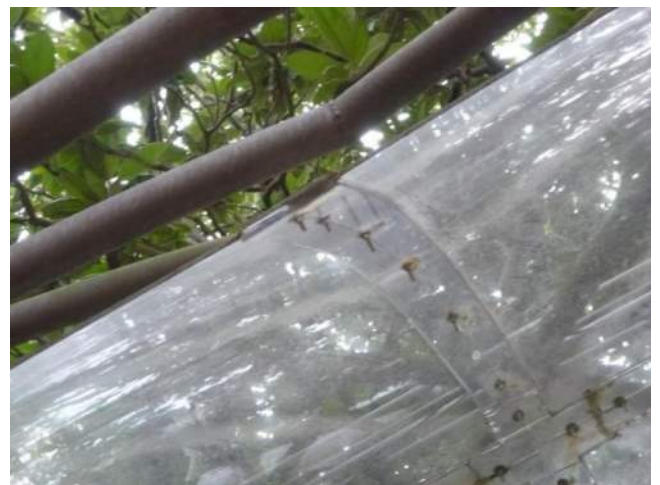
Figure 7.2-64. View of a typical joint in the polycarbonate sheathing of the canopy structure.
