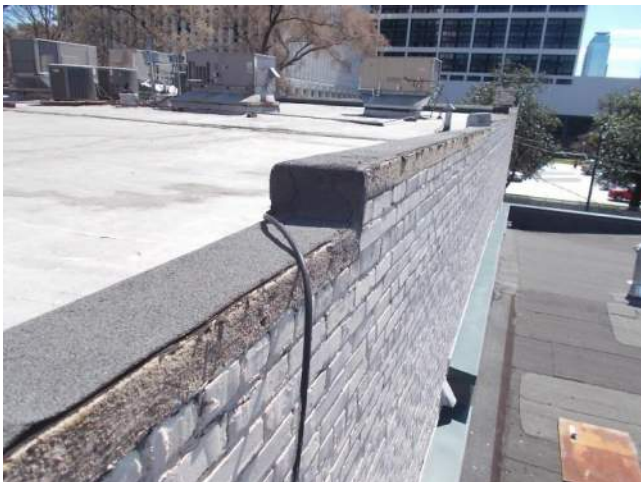
Figure 6.3-9. GSMB base flashings extend onto the horizontal surface of the stone copings.
