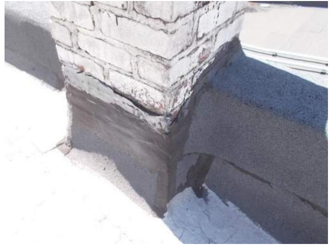
Figure 6.3-12. Roof membrane contained liquid membrane along the terminating edge of the membrane.
