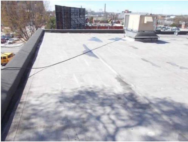
Figure 6.3-5. View of the main lower roof area from the northwest and southeast corner of the roof.
