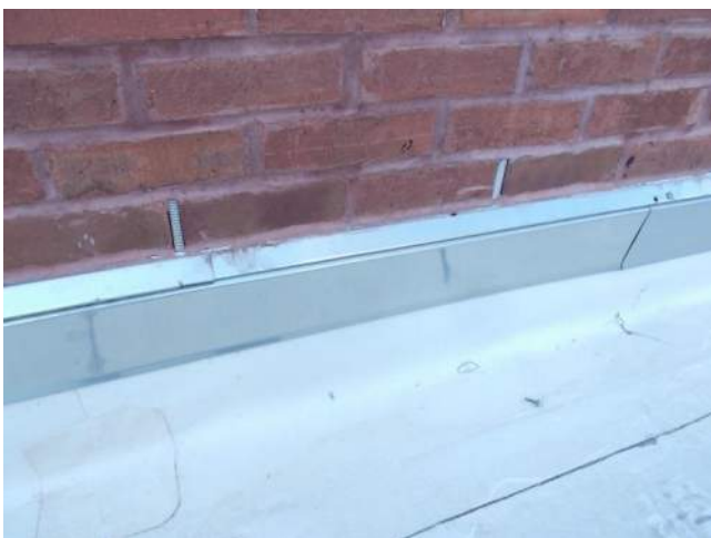
Figure 3.1-19. Roof termination on the connector roof integrated with a through wall flashing and weeps.
