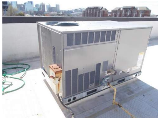
Figure 5.5-4. View of an RTU on the upper roof of the Pritchett Center.
