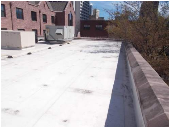
Figure 5.1-1. Overall view of the main lower roof area looking from the southwest corner of the roof.
