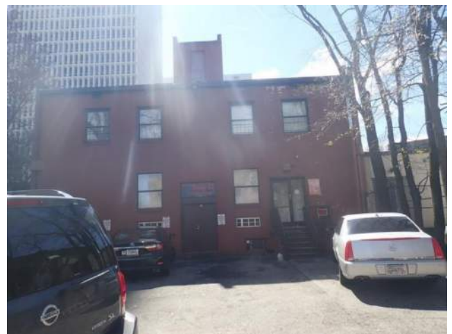
North facade of Tate Hall.
