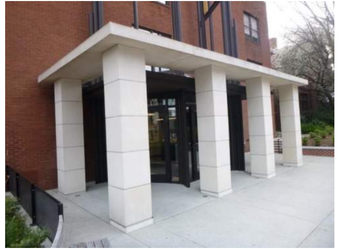
Figure 4.2-18. View of the cast stone covered entrance portico on the south elevation.
