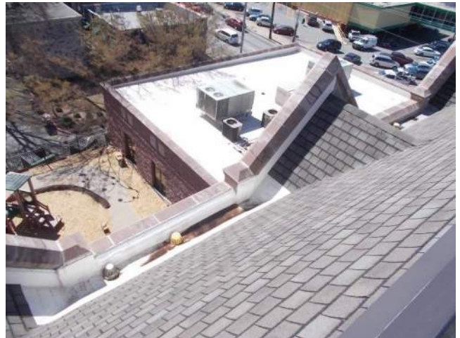
Figure 5.1-18. Overall view of the main upper roof area.
