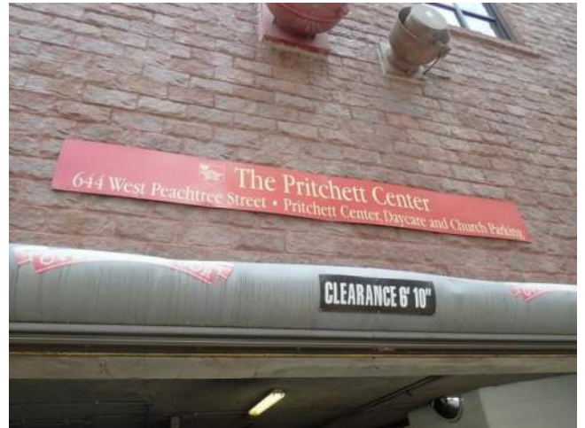
Figure 5.3-4. View of an overhead door at the upper level entrance of the Pritchett center parking structure.
