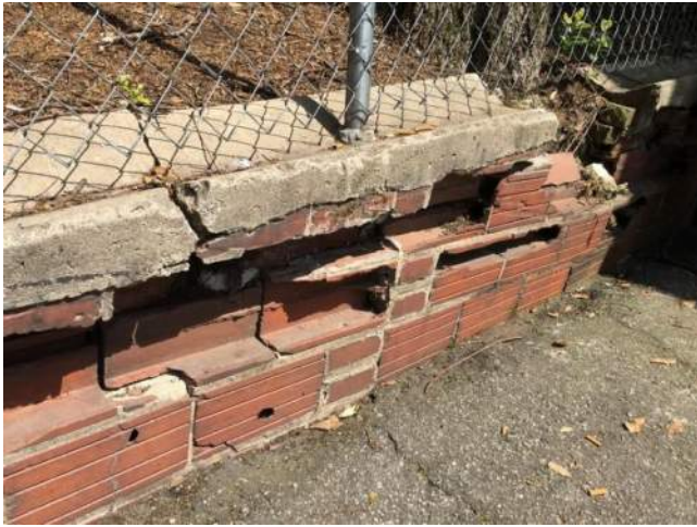
Figure 7.3-5. View of the hollow brick masonry tile retaining wall at the rear entrance drive.
