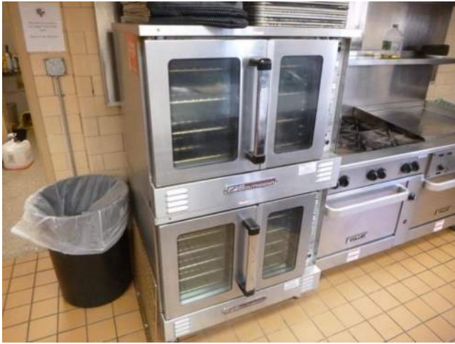
Figure 4.3-9. View of the double oven in the Parish House kitchen.
