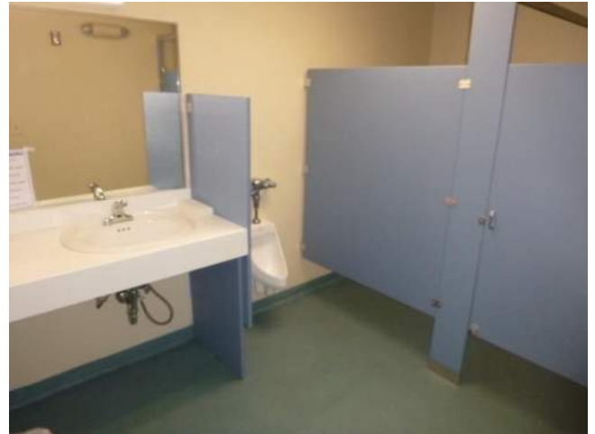
Figure 5.4-10. View of a typical restroom on the second floor.
