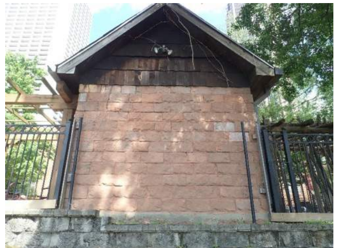
Figure 7.5-4 View of the stone masonry storage shed at the playground area.
