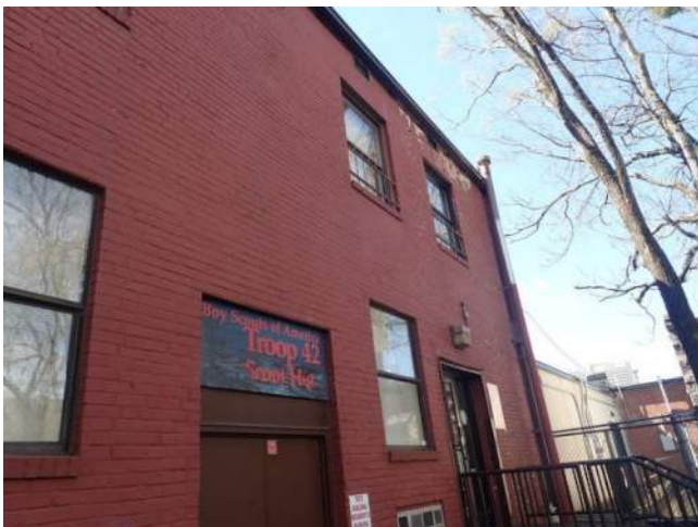
Figure 6.4-7. The brick masonry at Tate Hall was painted at the north, east, and west facades.
