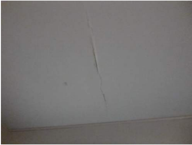
Figure 6.5-7. View of typical condition of finishes on the interior of Tate Hall.
