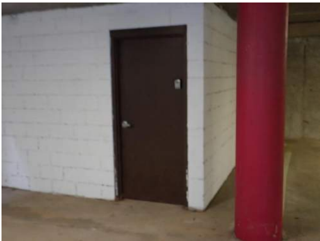
Figure 5.3-15. View of a typical storage space at the corner of the Pritchett center parking structure.
