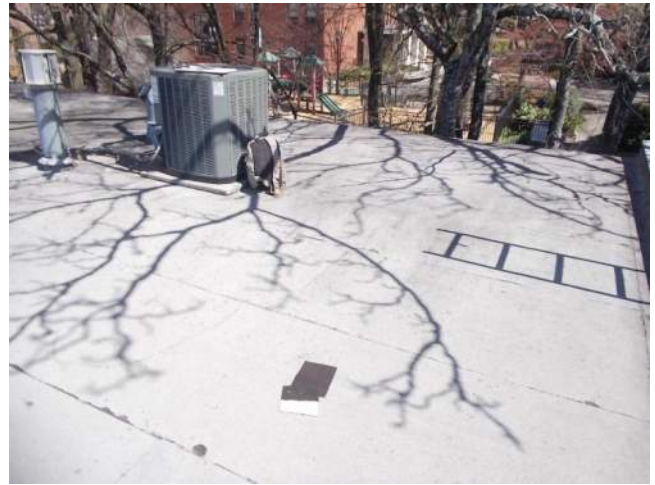
Figure 6.1-2. Overall view of the roof.
