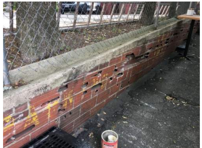
Figure 7.3-4. View of the hollow brick masonry tile retaining wall at the rear entrance drive.
