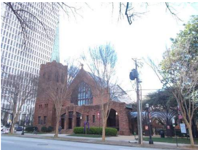
East facade of the Church and Chapel Building.
