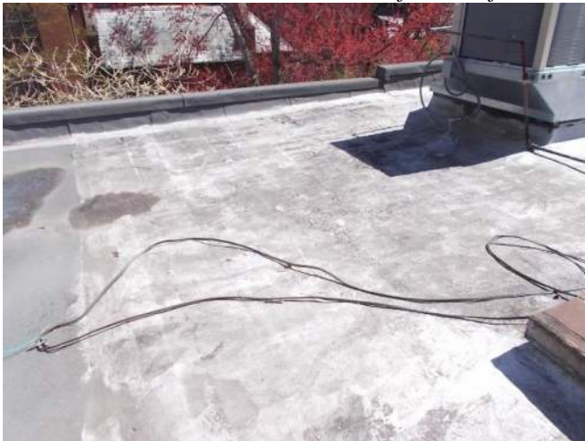
Figure 6.3-7. Weathered, deteriorated, and faded aluminum coating.
