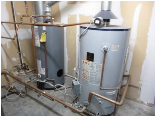
Figure 5.5-9. View of hot water heaters in a mechanical closet on the third floor of the Pritchett Center.
