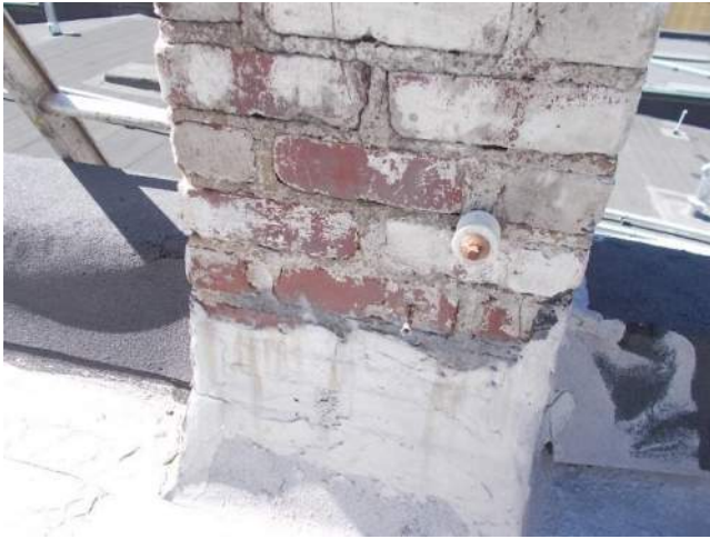
Figure 6.3-11. Roof membrane terminated onto the face of the brick masonry piers.
