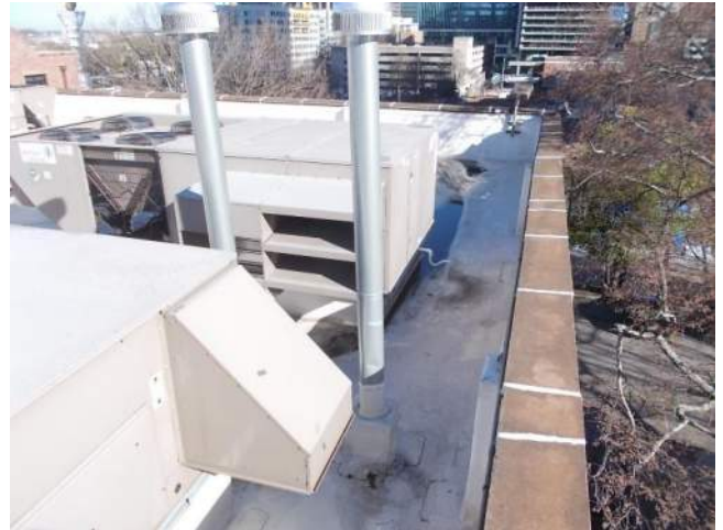
Figure 4.1-4. Overall view of the roof looking from the top of the west parapet wall.
