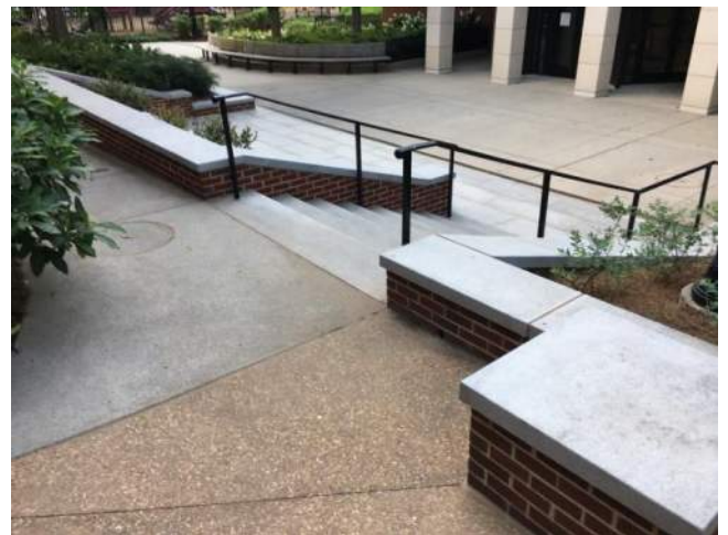
Figure 7.3-8. Partial view of a site wall at the Kennedy Commons Courtyard.
