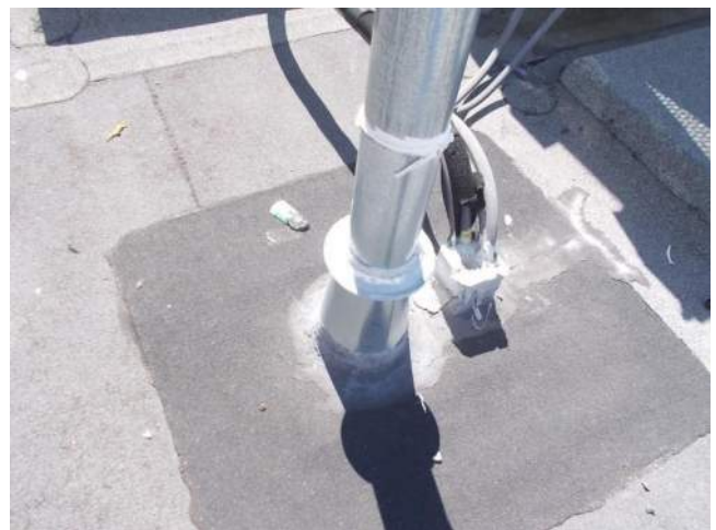
Figure 6.2B-6. Penetration with liquid membrane seals in good condition.
