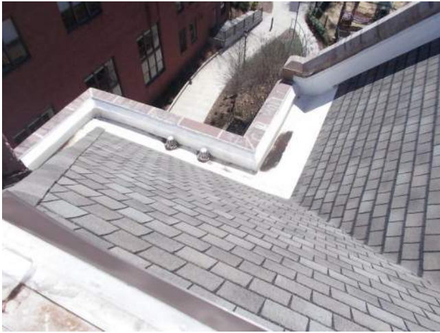
Figure 5.1-15. Overall view of the main upper roof area.
