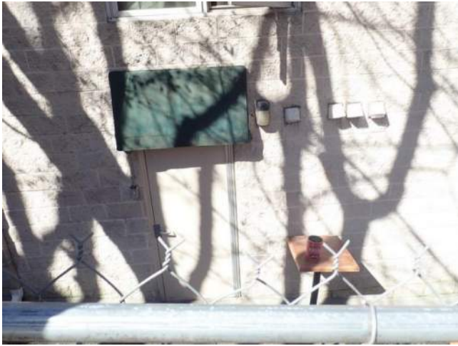
Figure 6.4-3. Surface mounted awnings were installed over entrance doors at the first floor of the building.
