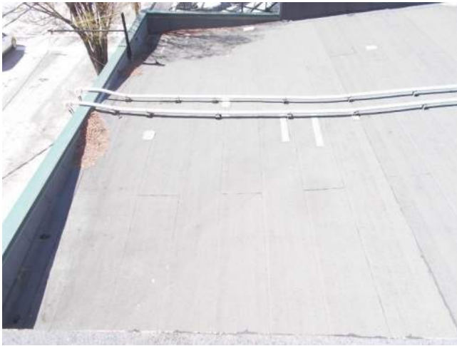
Figure 6.2D-1. Overall view of the roof area.
