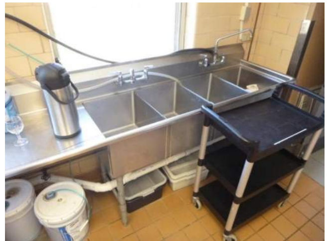
Figure 4.3-12. View of well sinks in the Parish House kitchen.
