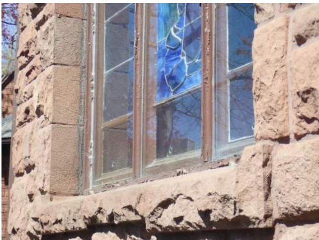
Figure 2.2-23. Deteriorated wood trim with failed coating.
