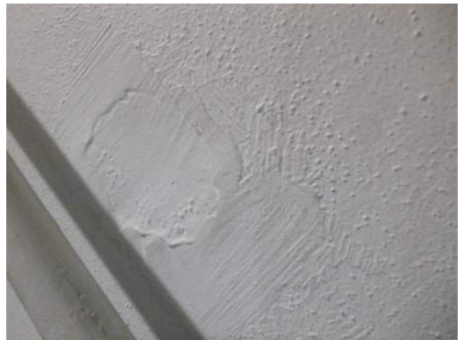
Figure 6.5-10. View of patch repair on a wall in Tate Hall.
