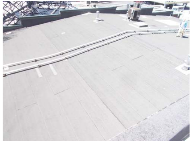
Figure 6.2D-2. Overall view of the roof area.
