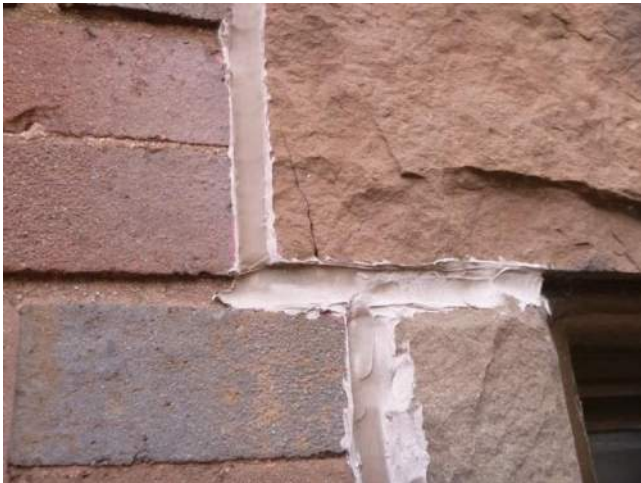
Figure 3.2-15. View of sealant repairs at joints at stone window surrounds.
