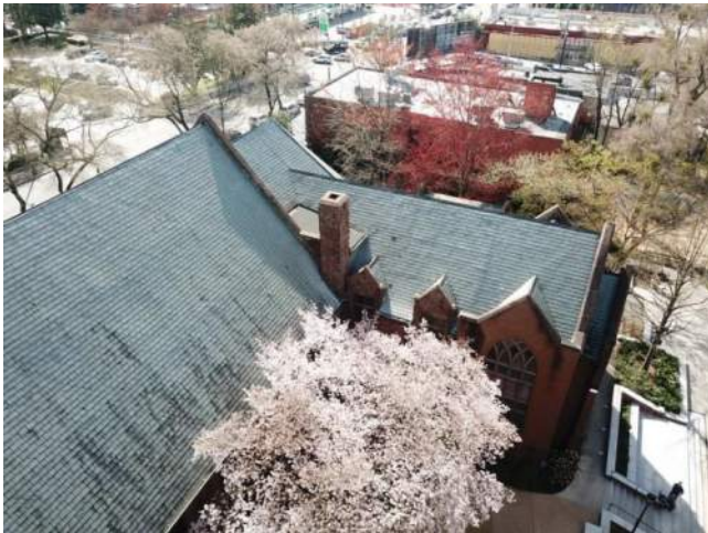
Figure 2.1-5. Overall view of the Church and Chapel roofs from our drone survey.
