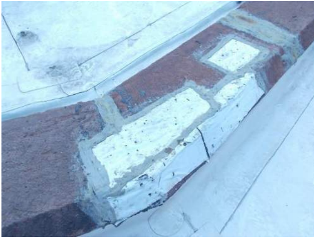
Figure 3.1-15. Self-adhered membrane and sealant repairs on the terra cotta coping units.
