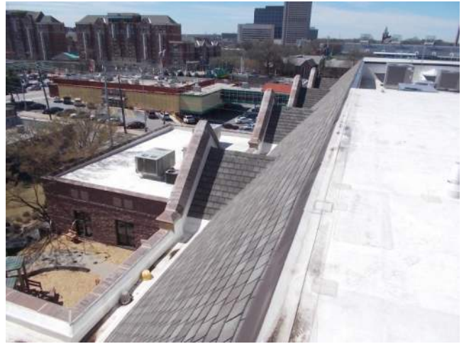
Figure 5.1-16. Overall view of the main upper roof area.
