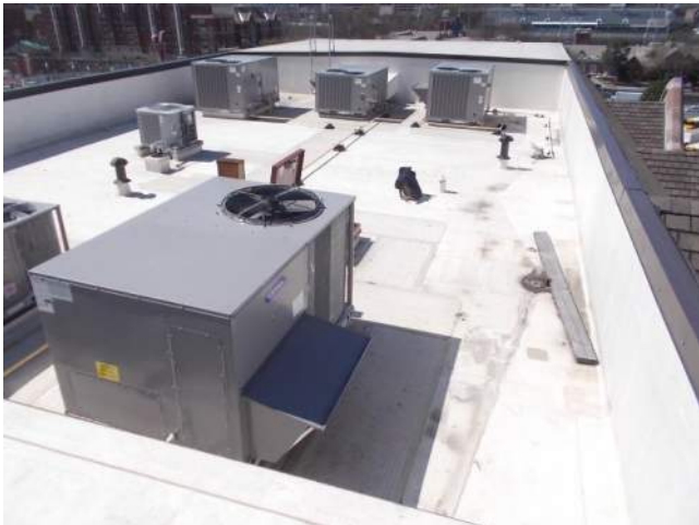
Figure 5.1-17. Overall view of the main upper roof area.
