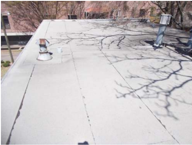
Figure 6.1-1. Overall view of the roof.
