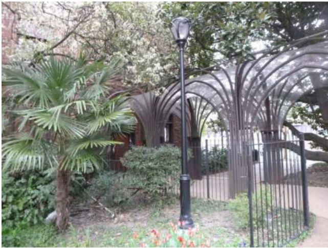
Figure 7.2-1. Partial view of the covered walkway and canopy structure.
