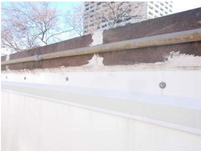
Figure 4.1-7. Surface mounted, metal counter flashing just beneath the roof coping.
