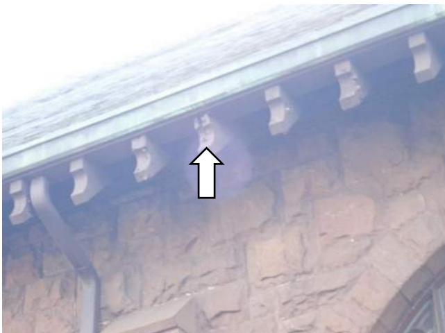
Figure 2.2-29. View of a split rafter tail on the Church Building.
