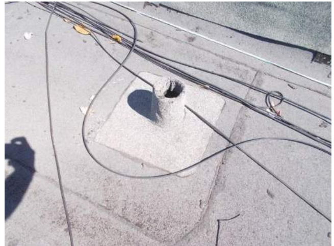
Figure 6.2B-4. Liquid membrane patch on the roof area in good condition.
