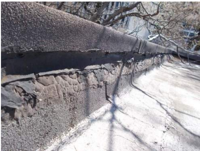
Figure 6.3-15. Liquid membrane and sealant installed between the GSMB base flashing and cap flashing.
