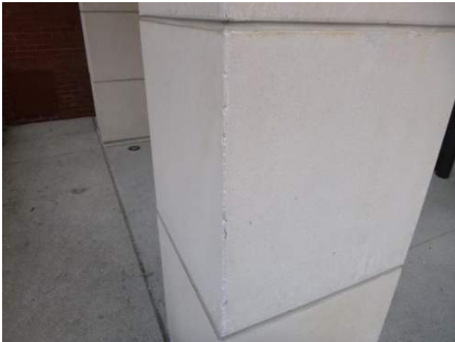
Figure 4.2-19. Partial view of a typical cast stone column.
