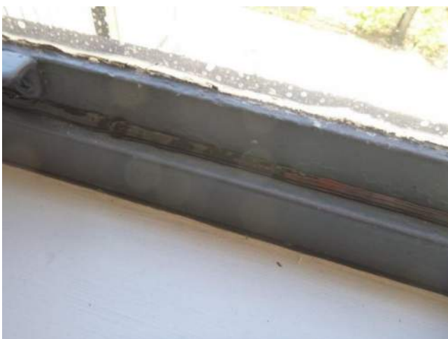
Figure 4.3-7. View of a typical sealed window in Ellis Hall in the Parish House.
