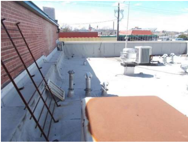
Figure 6.2B-1. Overall view of the roof area looking from the southeast corner of the roof.
