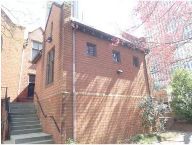
Figure 2.2-19. No deficiencies in the block bond masonry veneer at the Chapel Building.
