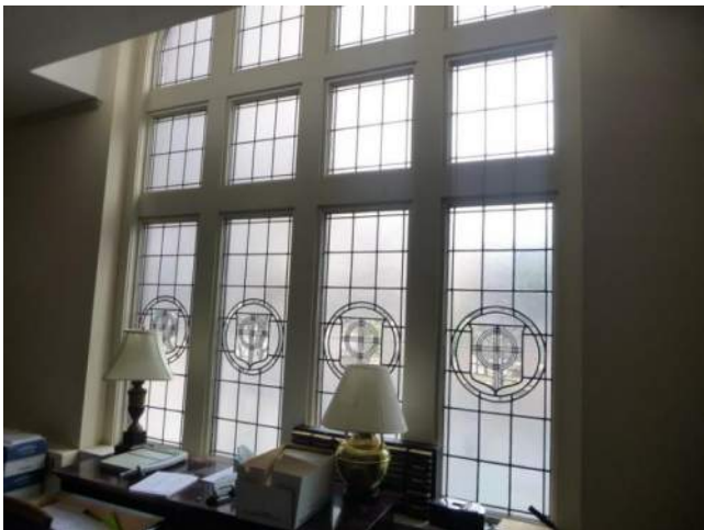
Figure 3.3-27. Overall view of the ganged leaded windows in the Horseshoe Room.
