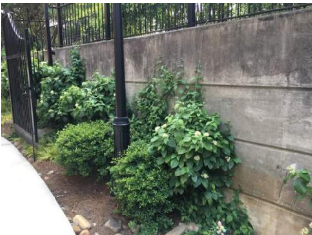
Figure 7.3-97. View of a concrete retaining wall adjacent to the Pritchett Center playground.
