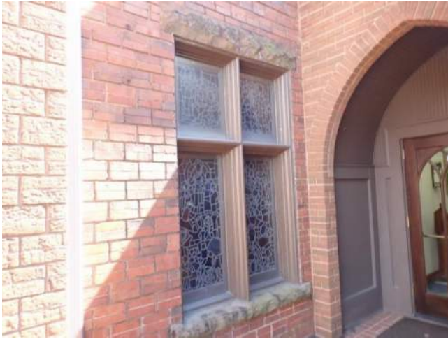
Figure 2.2-13. Brick masonry mass wall assembly laid in block bond with granite headers and sills.
