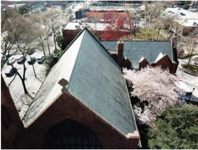
Figure 2.1-3. Overall view of the roofs of the Church and Chapel buildings.
