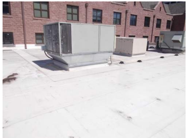
Figure 5.1-2. Overall view of the main lower roof area looking from the southwest corner of the roof.
