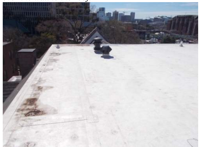
Figure 5.1-14. Overall view of the main upper roof area.
