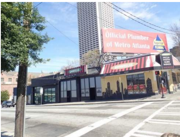
West facade of the restaurant/retail facade.
