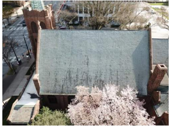
Figure 2.1-4. Overall view of the roof of the Church from our drone survey.
