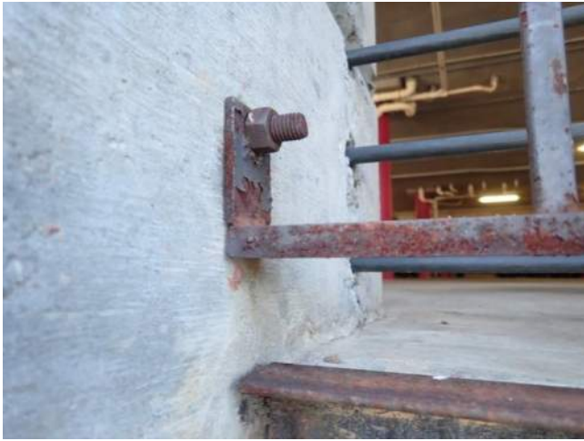
Figure 5.2-7. The fencing was bolted to the concrete structure.
