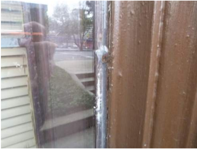
Figure 3.2-19. View of an acrylic panel fastened over the glass light to the wood window frame.
