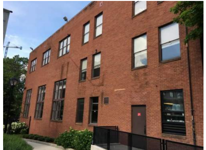
View of the west facade of the Parish House.
