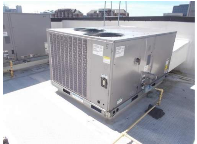
Figure 5.5-2. View of an RTU on the upper roof of the Pritchett Center.
