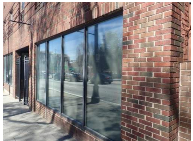
Figure 6.4-8. The masonry at the south elevation was uncoated.
