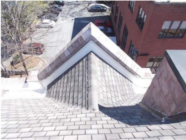
Figure 5.1-21. TPO membrane terminated under a metal counterflashing underneath the coping.
