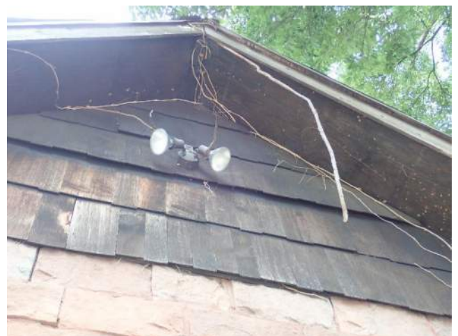
Figure 7.5-6. View of the wood eaves and shake cladding of the storage shed.
