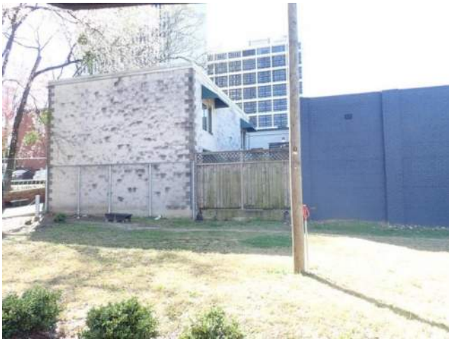
Figure 6.4-1. The facade of the Covenant Community building consists of split face CMU with vinyl window units and wood trim.
