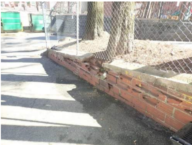
Figure 7.3-35. View of the hollow brick masonry tile retaining wall at the rear entrance drive.
