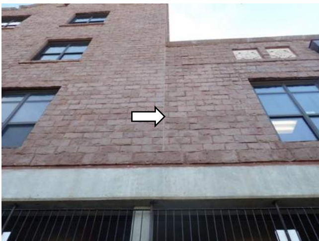
Figure 5.2-5. Vertical expansion joint at the transition between a three story and a one story structure at the west elevation.
