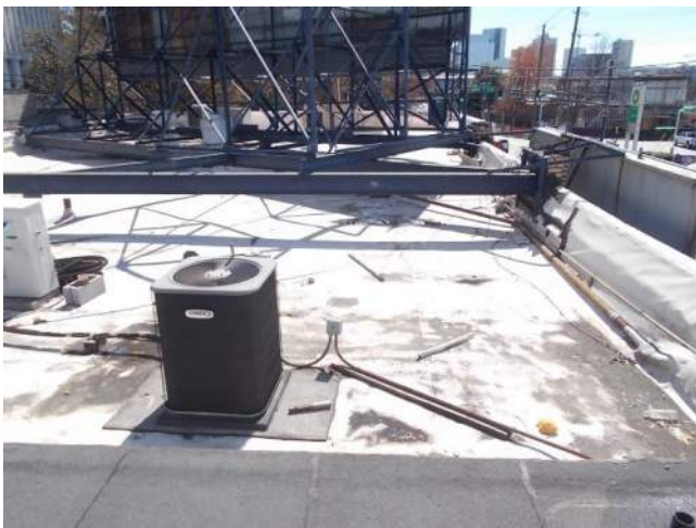
Figure 6.2C-1. Overall view of the Roof Area C.
