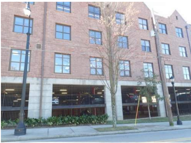
Figure 5.2-11. No deficiencies on exposed cast-in-place concrete elements at the parking garage.
