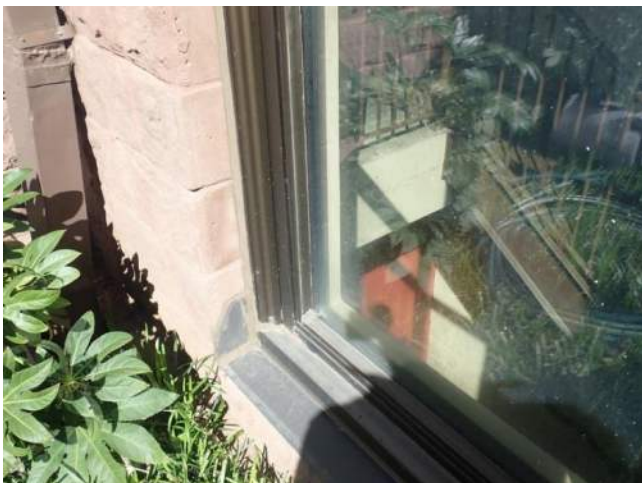
Figure 5.2-17. The window perimeter sealants were in good condition.
