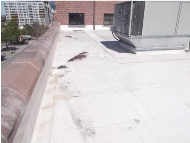
Figure 5.1-3. Overall view of the main lower roof area looking from the southwest corner of the roof.
