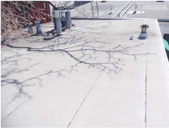
Figure 6.1-3. Overall view of the roof.
