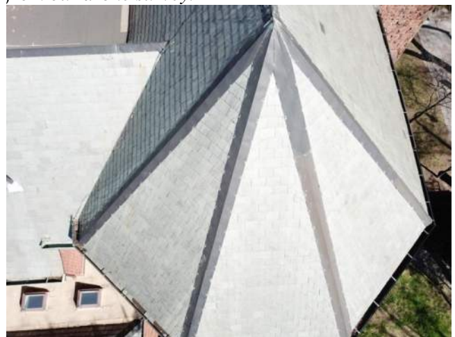
Figure 2.1-8. Overall view of the roof from our drone survey.
