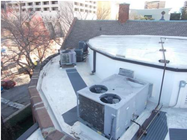
Figure 3.1-5. Partial view of the roof from the top of the east parapet wall of the Parish House roof.
