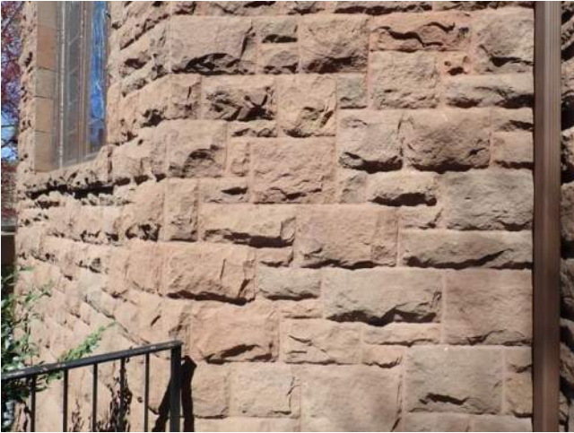
Figure 2.2-1. The sandstone masonry was observed to be structurally sound.
