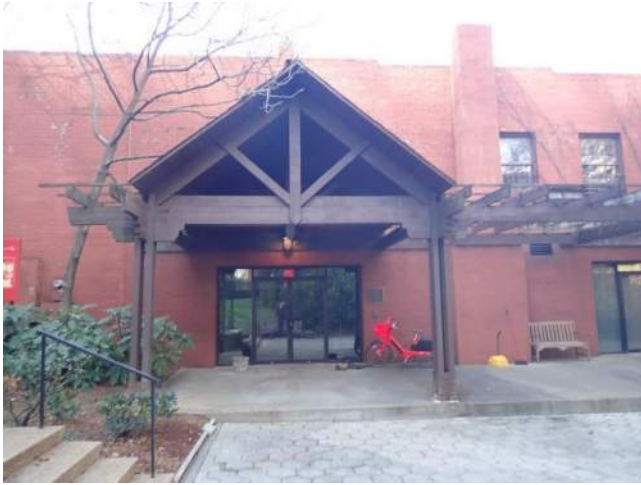
Figure 6.4-15. A painted, wood framed pergola and entrance canopy with asphalt shingle roofing is attached to the east facade.
