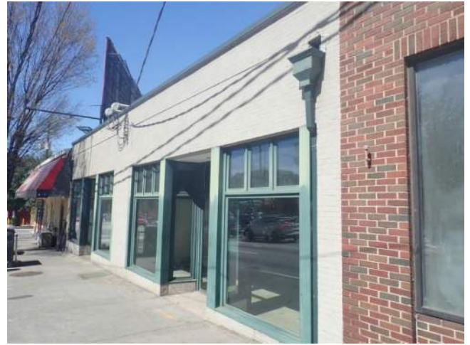
Figure 6.4-4. Street facing facades are painted brick masonry with aluminum storefront window systems.
