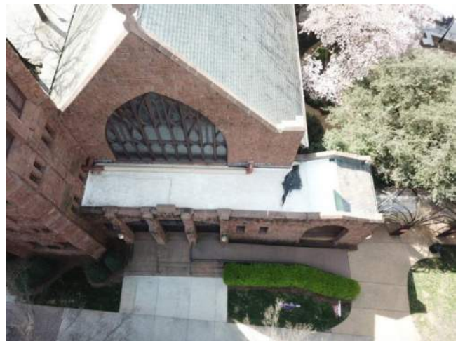
Figure 2.1-2. View of the West Peachtree Street entrance roof from our drone survey.
