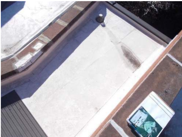
Figure 3.1-1. Overall view of the south end of the lower roof from the top of the east parapet wall of the Parish House roof.
