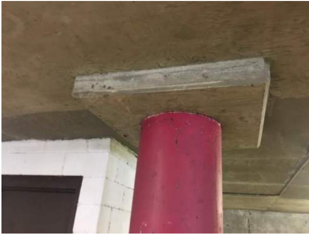
Figure 5.3-1. View of a typical concrete column and drop panel.
