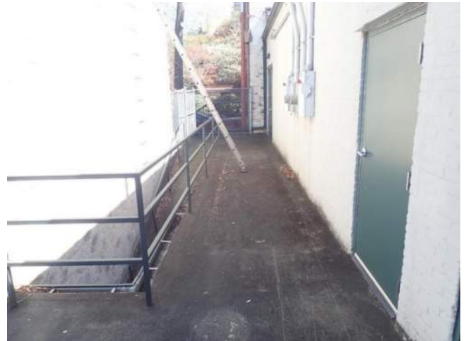
Figure 6.4-6. Rear facades of the spaces are also coated with a similar material.
