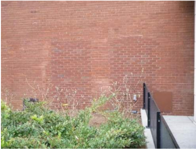
Figure 4.2-5. View of areas of masonry fill at previous openings on the south facade.
