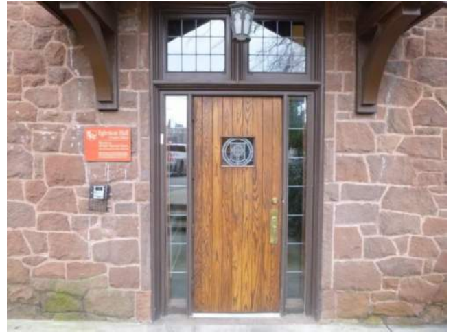
Figure 3.2-20. View of the covered entrance door on the north elevation of the Egleston building.
