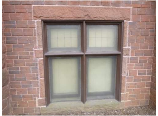
Figure 3.2-14. View of sealant repairs between the brick masonry and stone window surrounds.
