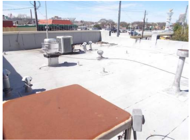
Figure 6.2A-2. Overall view of the roof area looking from the southeast corner of the roof.
