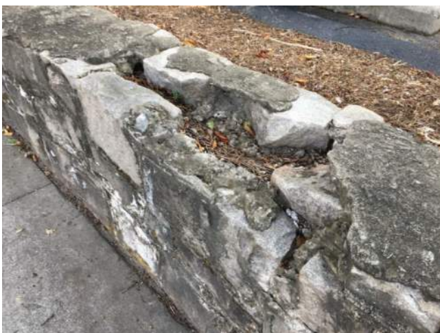
Figure 7.3-15 View of the stone retaining wall on Ponce De Leon Avenue.
