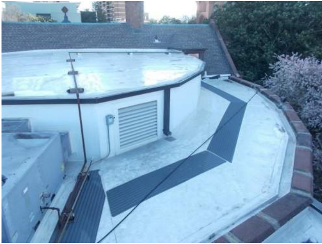
Figure 3.1-3. Partial view of the roof from the top of the east parapet wall of the Parish House roof.
