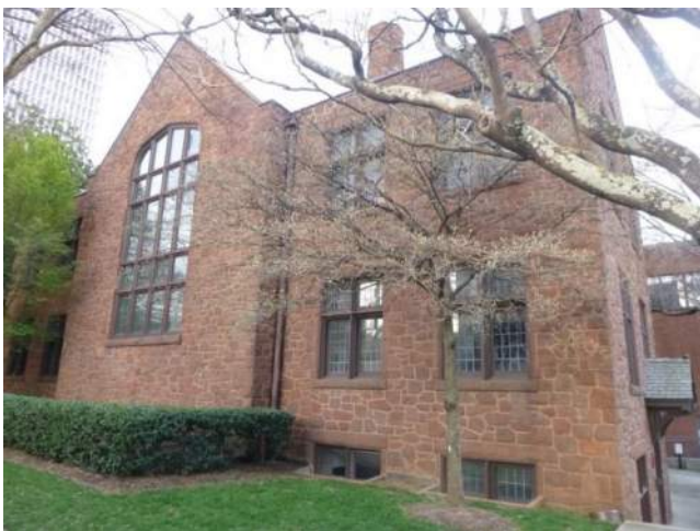
Partial east facade of Egleston Hall.
