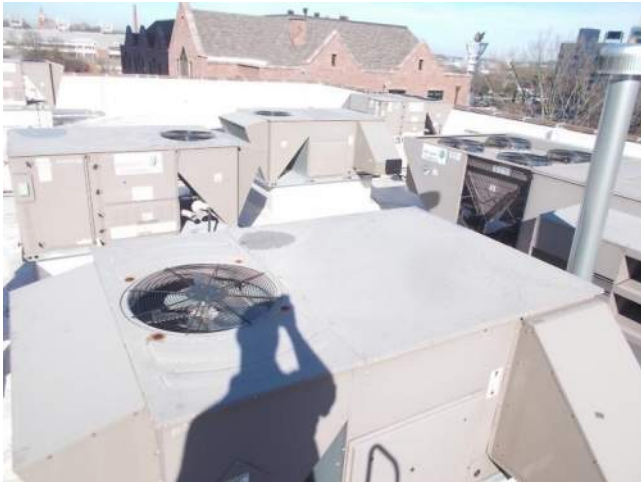
Figure 4.1-3. Overall view of the roof looking from the top of the west parapet wall.
