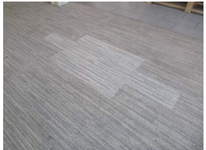
Figure 4.3-6. View of a section of replaced carpet tile in Ellis Hall.
