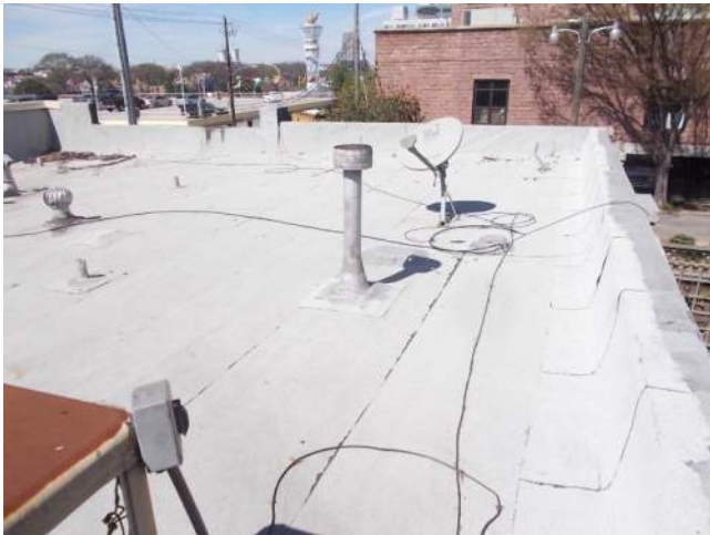
Figure 6.2A-3. Overall view of the roof area looking from the southeast corner of the roof.
