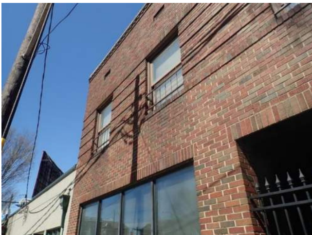
Figure 6.4-13. Aluminum framed window systems at the north elevation and at the second floor of the south and east elevations.
