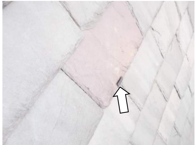
Figure 3.1-6. Copper clips along the bottom edge of a replaced shingle.
