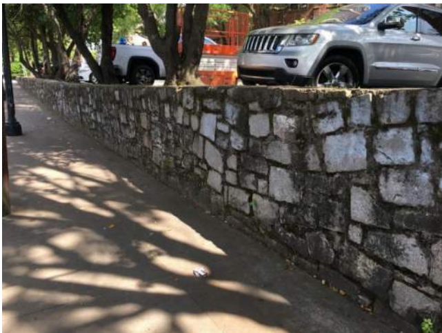
Figure 7.3-13 View of the stone retaining wall on Ponce De Leon Avenue.
