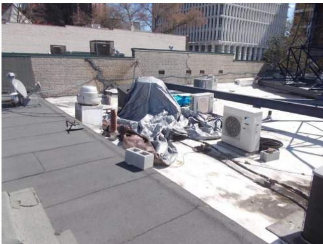
Figure 6.2C-3. Overall view of the Roof Area C.
