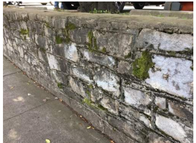
Figure. 7.3-149. View of the stone retaining wall on Ponce De Leon Avenue.
