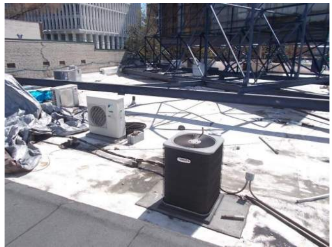
Figure 6.2C-2. Overall view of the Roof Area C.
