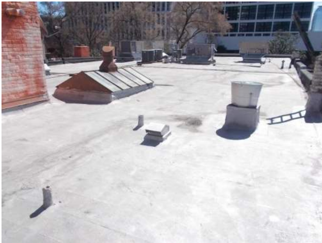
Figure 6.3-1. View of the main lower roof area from the northwest and southeast corner of the roof.
