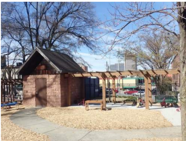
Figure 7.5-3. Overall view of the storage shed and wood pergola structure.
