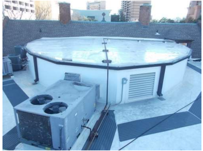
Figure 3.1-4. Partial view of the roof from the top of the east parapet wall of the Parish House roof.
