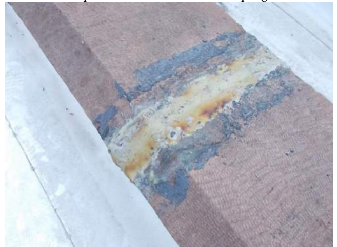
Figure 3.1-14. View of numerous layers of sealants at a coping joint.
