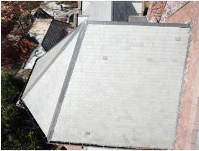
Figure 2.1-9. Overall view of the roof from our drone survey.
