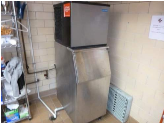
Figure 4.3-11. View of the standalone ice maker in the Parish House kitchen.
