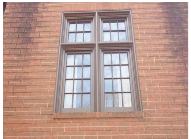
Figure 2.2-24. The wood framed window systems within the Chapel addition were in good condition.
