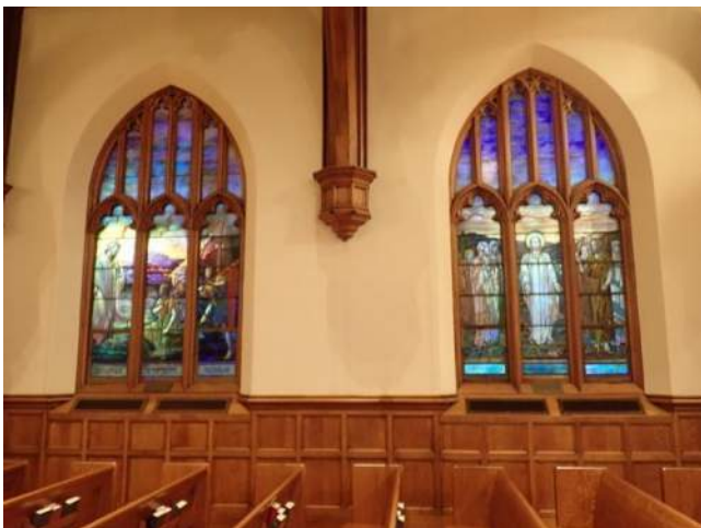
Figure 2.3-9. View of typical stained glass windows at the Nave aisle.
