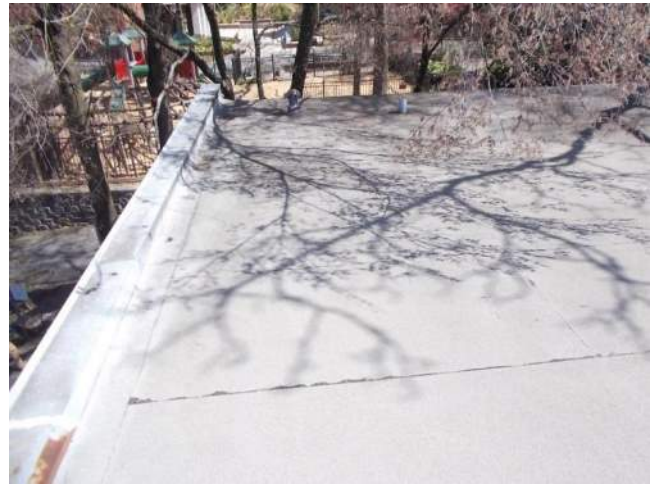
Figure 6.1-4. Overall view of the roof.
