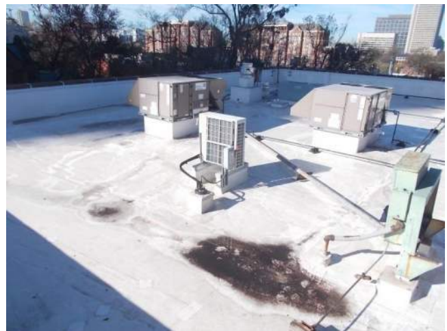
Figure 4.1-2. Overall view of the roof looking from the top of the west parapet wall.
