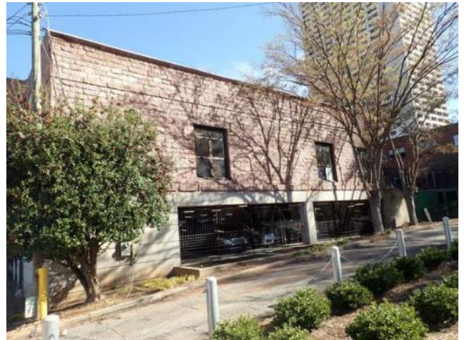
Figure 5.2-4. Overall view of the condition of the manufactured stone masonry facade.
