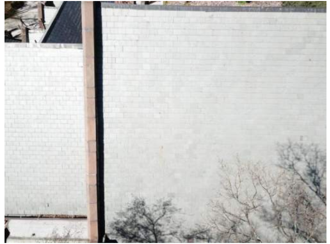
Figure 2.1-10. Overall view of the roof from our drone survey.
