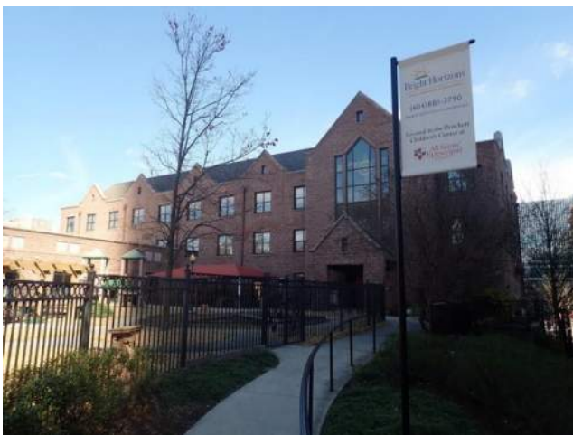
South facade of the Pritchett Children's Center
