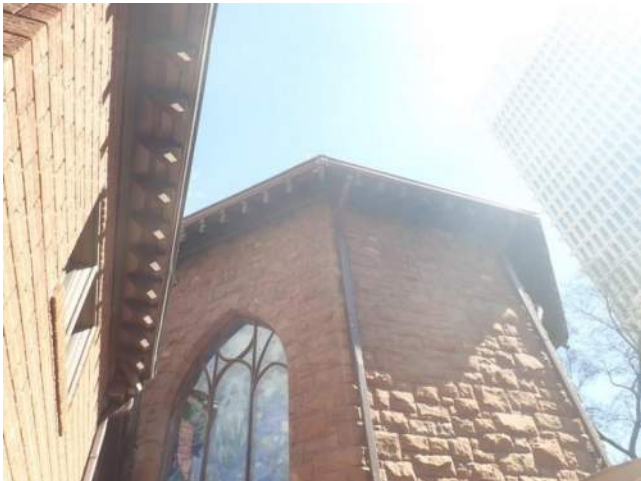
Figure 2.2-27. Decorative wood rafter tails and vented wood soffits beneath the overhanging steep slope slate shingle roof areas.
