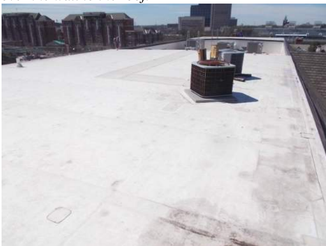
Figure 5.1-13. Overall view of the main upper roof area.
