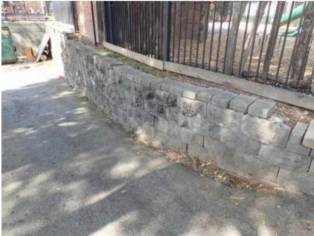
Figure 7.3-11 View of the segmental retaining wall at the west end of the property.
