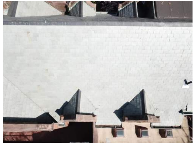
Figure 2.1-6. Overall view of the Chapel addition roof from our drone survey.
