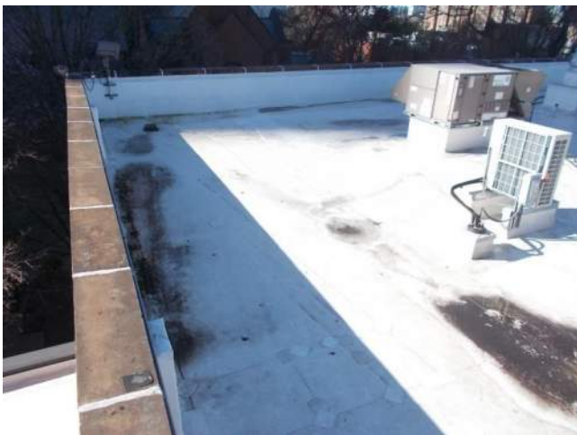
Figure 4.1-1. Overall view of the roof looking from the top of the west parapet wall.
