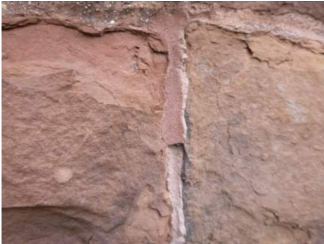
Figure 3.2-7. View of a previous repointing and colored mortar on the Egleston building.
