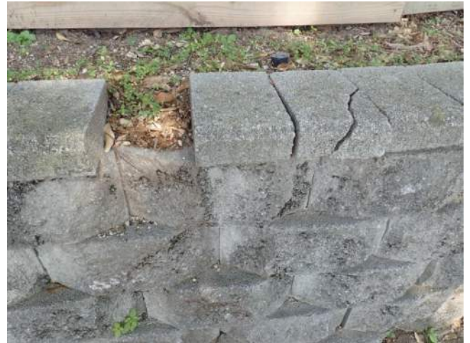
Figure. 7.3-128. View of the segmental retaining wall at the west end of the property.
