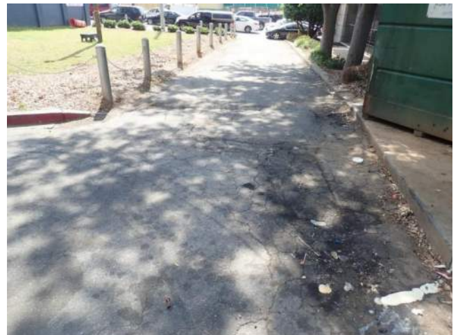
Figure 7.4-410. View of the rear entrance drive near the covenant community church.
