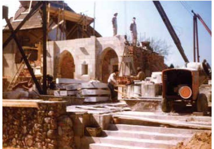
Construction of Cloister
