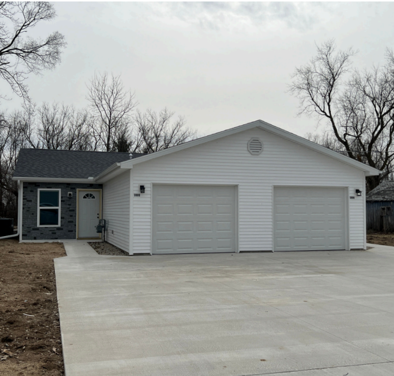
Duplex units in the Village of Rosebush, Isabella County, that received funding from the MSHDA MI Neighborhood program in 2025.
