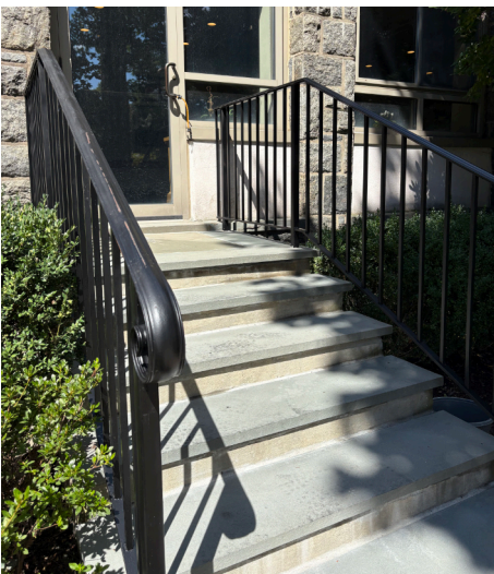
Westminister's stairs were repaired!
