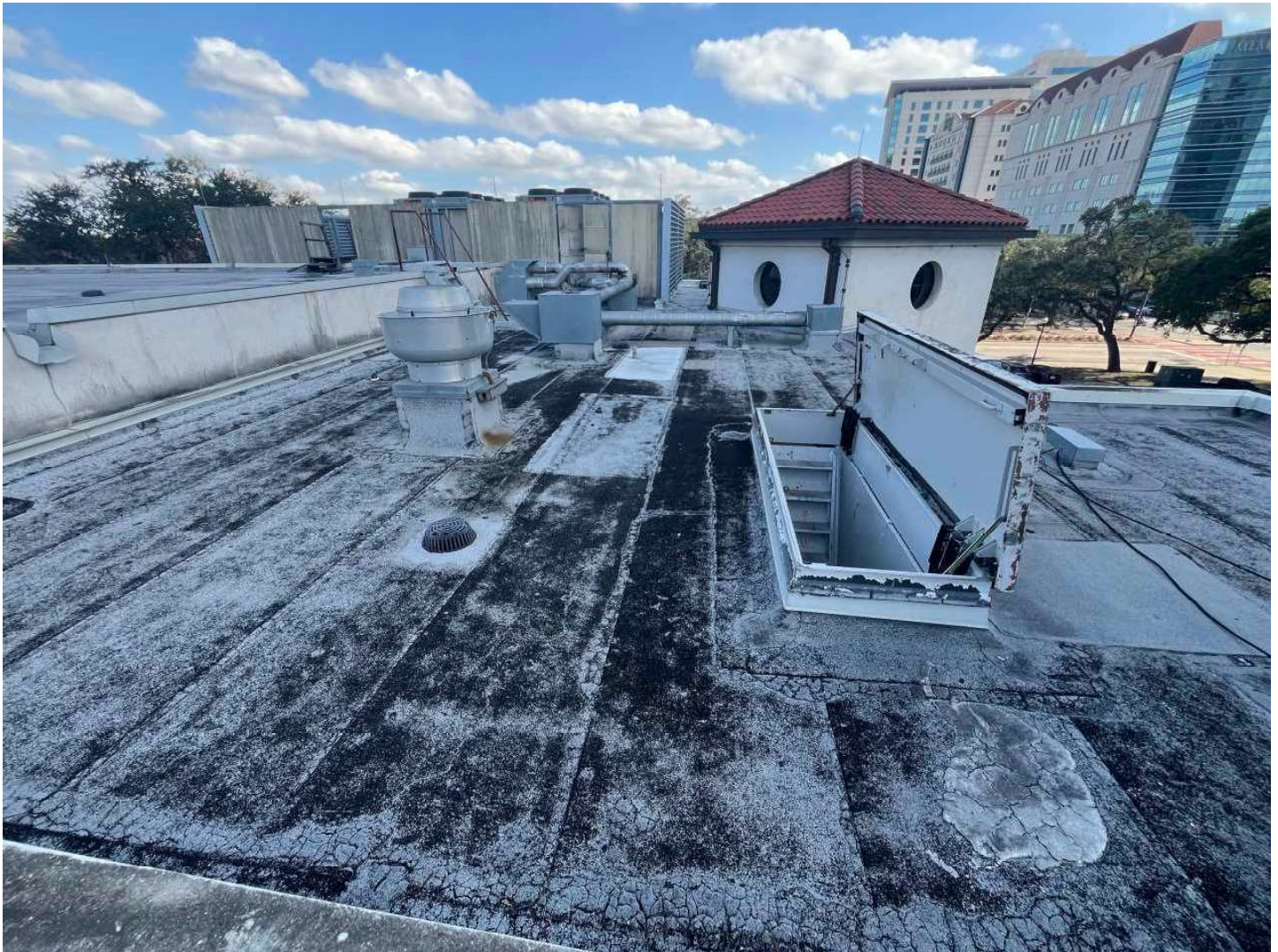
35 35-IMG_6162 Date Taken: 2/7/2025 Section A Roof - Roll Roofing needs to be replaced
