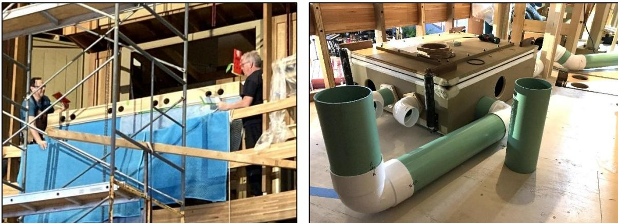
Nordlie craftsmen worked with RLC volunteers December 2-4 to place a large windchest in the Great Division, a refurbished windchest from the Holtkamp organ and several wind “reservoirs” or bellows. The reservoirs were connected to the wind trunks previously installed in the loft floor using 4- and 6-inch PVC pipe.
