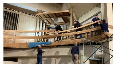
It is exciting to see the transformation in the pipe loft! The Swell Division is enclosed on the east wall, the center Choir Division is framed, and more curved oak casework is up. Once the infrastructure is complete, organ builder J.F. Nordlie will start setting pipes.
