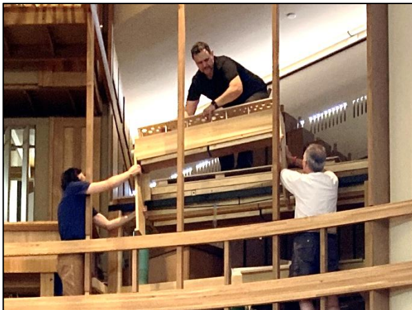
Another small off-set windchest and toe board guided into place.
