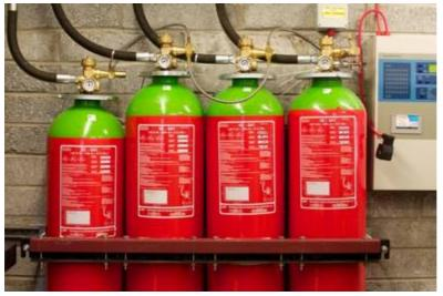
IG-541 is an inert gas which is also commonly known by the brand name INERGEN. The composition of the gas is 50% Nitrogen, 42% Argon and 8% Carbon Dioxide the green house effect and ozone depletion characteristic of the gas is nil. The gas is chemically inert, colourless, odourless, flavourless, non conductive and non corrosive. At normal temperatures it may be freely used with such materials as nickel, stainless steel, copper, brass, bronze and plastics.
