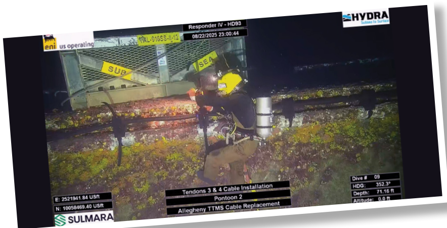
Fig. 2 – Gilbert installing a tendon tension monitoring system (TTMS) cables on the Allegheny Tension Leg Platform in Green Canyon Block 254 (GC-254) in the Gulf of Mexico.
